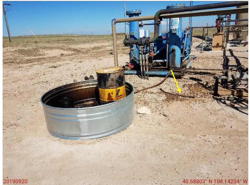
Photo 4: Photo taken from the north end of the location. Photo shows containers have been placed in secondary containment. Photo also shows stained soils observed in previous inspections have not been sufficiently cleaned/treated and/or removed.
