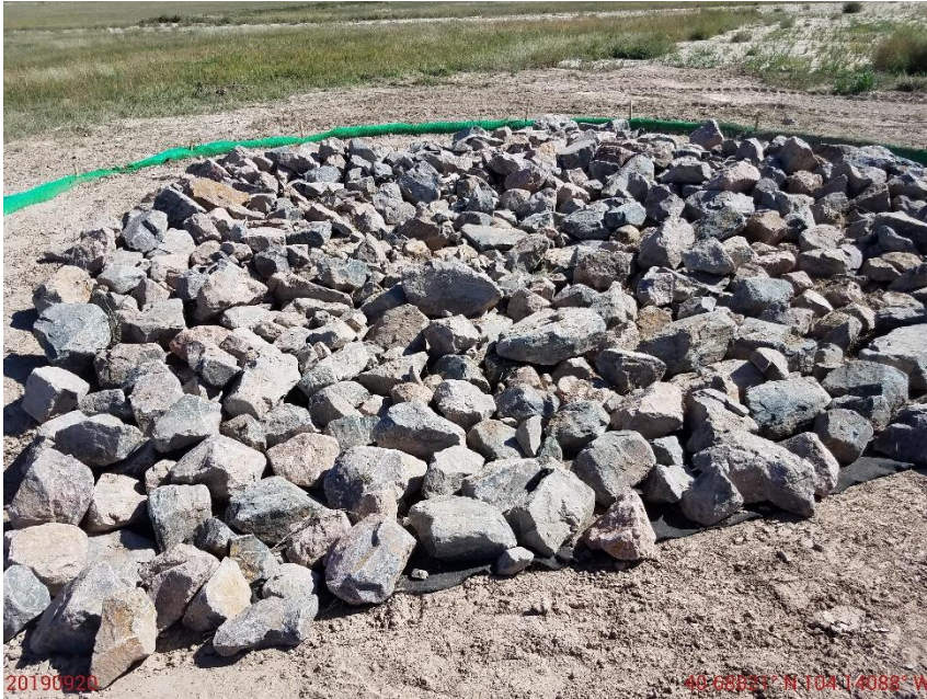
Photo 15: Photo taken from the northeast end of the location. Photo shows operator appears to have installed a sediment trap. BMP appears to be sufficient and proper functioning condition to meet the site's conditions post interim reclamation.
