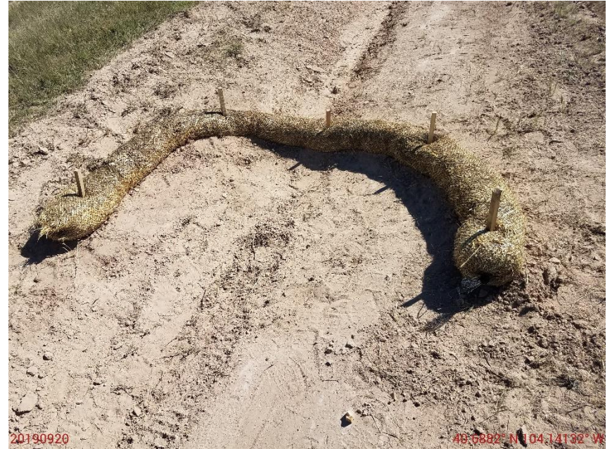
Photo 14: Photo of wattles within ditch. BMP appears to have been installed in accordance with good engineering practices.
