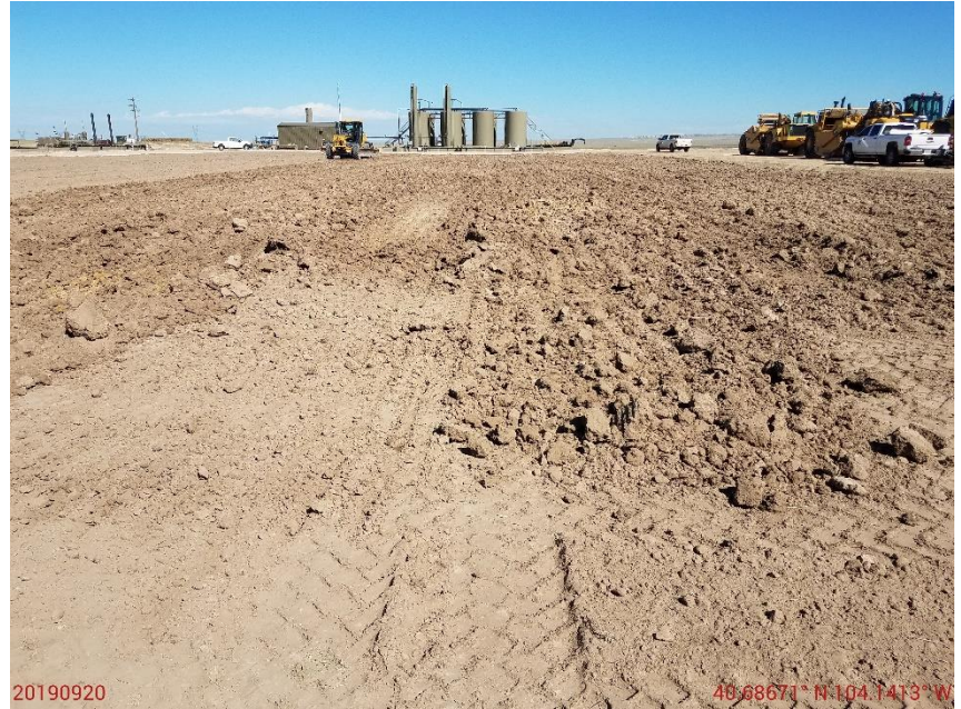
Photo 18: Photo taken from the south end of the location, facing north. Photo shows compaction alleviation in process. Rule 1003.c requires locations to be cross-ripped to a minimum depth of 18 inches. Photo shows location has only been ripped once in one direction. Contractor on site stated that the location was not planned to be cross-ripped in accordance with 1003.c.
