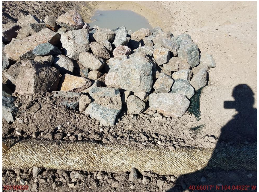
Photo 8: Photo taken from the outlet of the sediment trap on the north end of the location. Photo shows geotextile has been placed beneath the rip-rap of the outlet. Operator appears to have only used a single-type large aggregate within outlet
