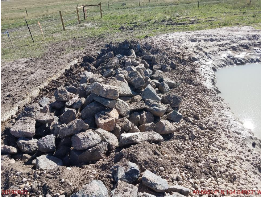
Photo 9: Photo of outlet at the sediment trap on the northeast end of the location. Operator appears to have installed outlet with a combination of sufficient, and appropriately sized (large/small) aggregate with a geotextile lining; Outlet appears to have been installed in accordance with good engineering practices.
