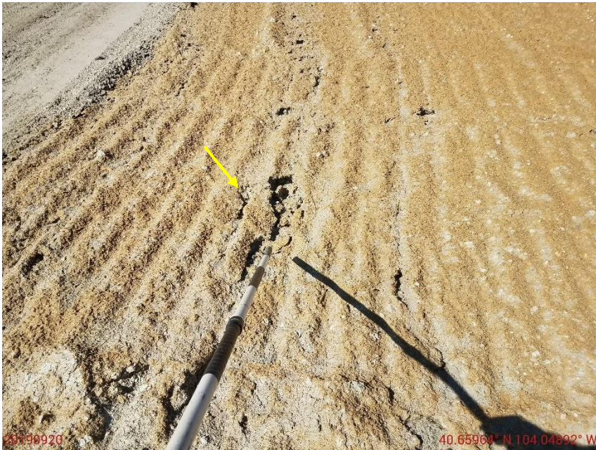
Photo 15: Continued from photo 14. Photo shows areas where operator tracked slope along the contour of the slopes, rather than up and down. As a result, rill erosion has formed on areas of the slopes
