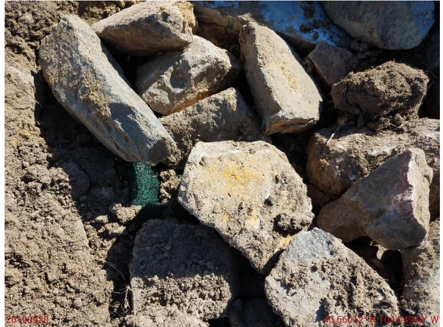
Photo 2: Continued from photo 1. Photo shows geotextile has not been placed under the rip-rap.
