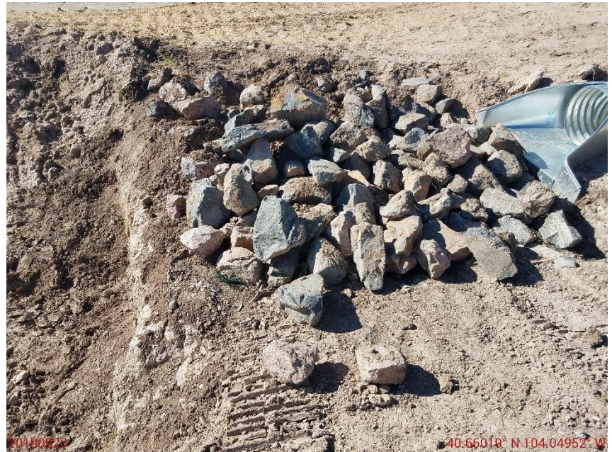
Photo 6: Photo taken from the sediment trap inlet on the south end of the location. Operator has placed geotextile under the rip-rap. Inlet has been constructed with a horizontal grade/cut without sufficient inlet/slope protections. This is not good engineering practices.
