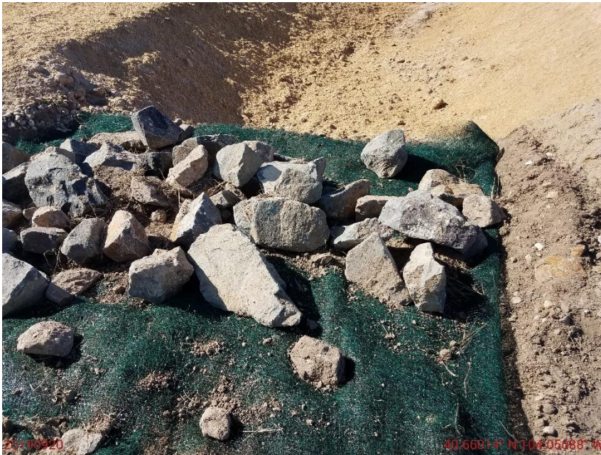
Photo 23: Continued from photo 22. Photo shows outlet has not been constructed in accordance with good engineering practices.
