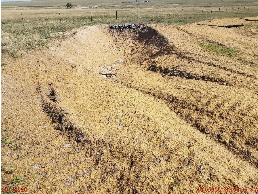
Photo 19: Photo taken from the sediment trap on the northwest corner of the location. Photo shows BMP has not been constructed in accordance with good engineering practices with sufficient inlet/outlet and slope protection. Photo shows erosion degradation evident at inlet.
