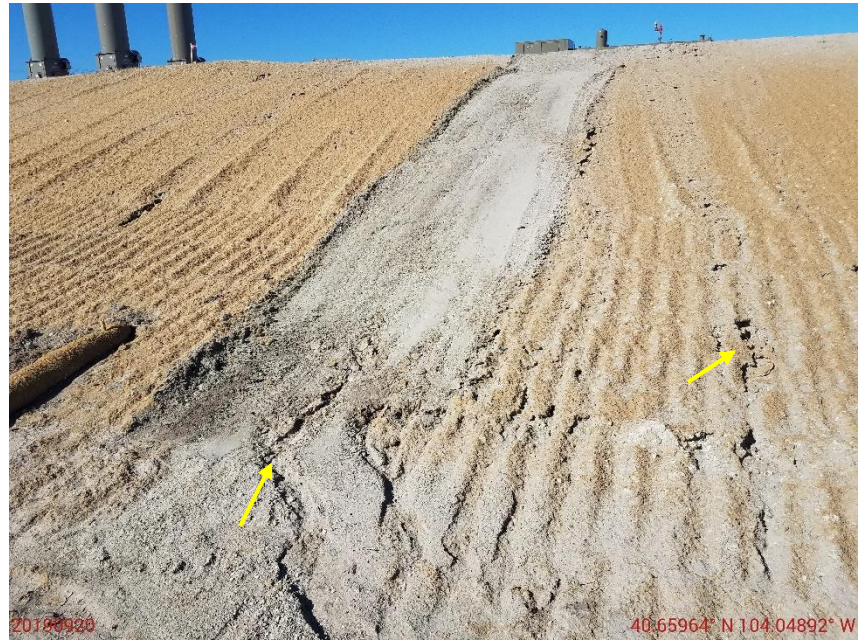
Photo 14: : Photo taken from the slopes on the east end of the location. Photo shows stormwater appears to have eroded the slopes of the location. Operator appears to have repaired erosion, however, it does not appear as though operator has installed BMPs to stabilize slope. Photo also shows areas where operator tracked slope along the contour of the slopes, rather than up and down. As a result, rill erosion has formed on areas of the slopes (arrow)
