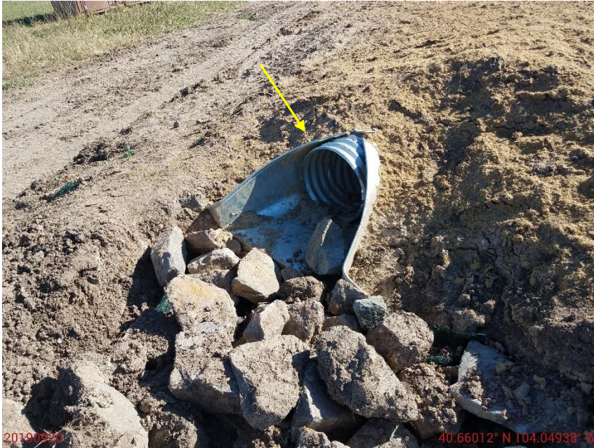
Photo 1: Photo taken from the culvert on the north end of the pad. Photo shows sufficient outlet protection has not been installed above culvert outlet.
