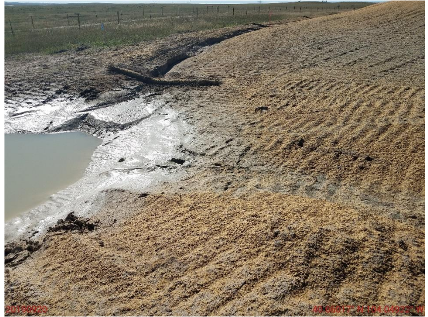
Photo 10: Photo of inlet at the sediment trap on the northeast end of the location, facing southeast. Photo shows BMP has not been constructed in accordance with good engineering practices and is missing sufficient inlet protections. Erosion degradation evident at inlet and diversion ditch. Additionally, operator appears to have installed a wattle at the inlet without repairing ditch.
