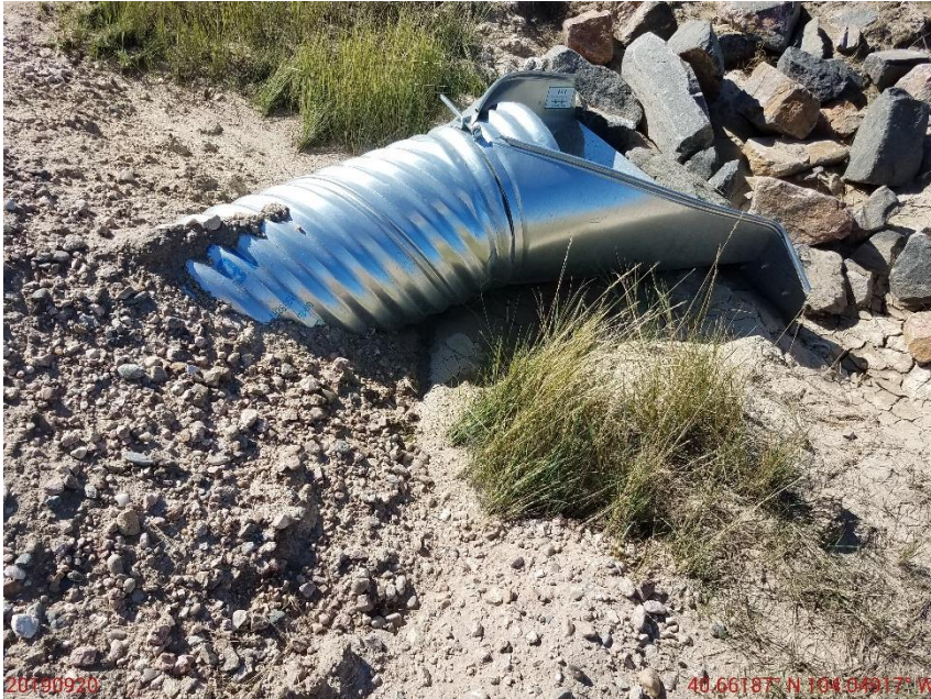
Photo 25: Photo taken from the culvert on the access road north of the pad. Photo shows sufficient outlet protection has not been installed above culvert outlet. Erosion degradation around culvert evident.
