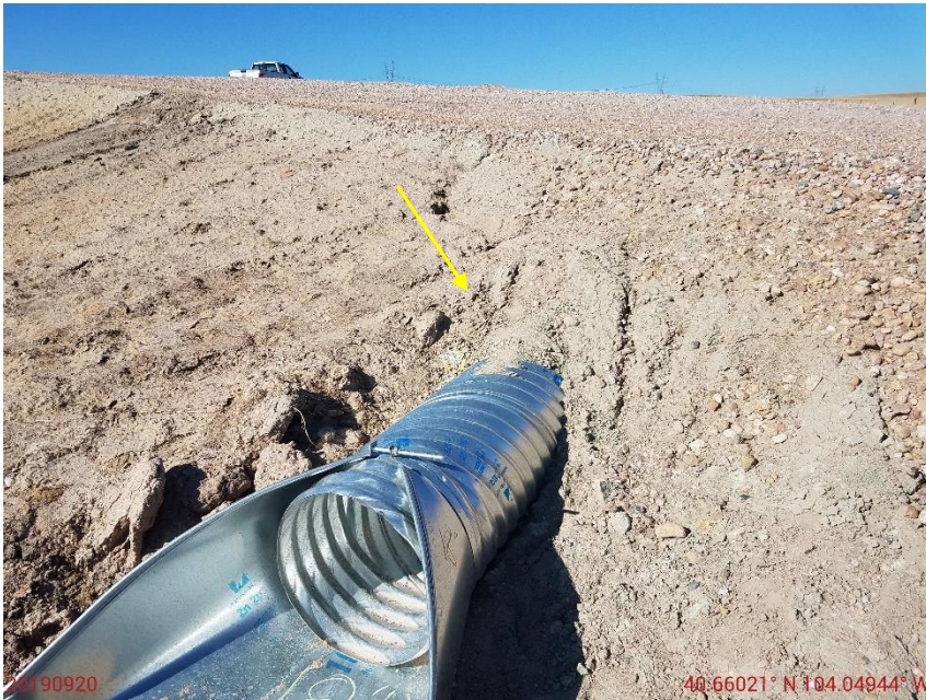
Photo 7: Photo taken from the culvert on the north end of the pad. Photo shows sufficient outlet protection has not been installed above culvert outlet. Erosion degradation around culvert evident.
