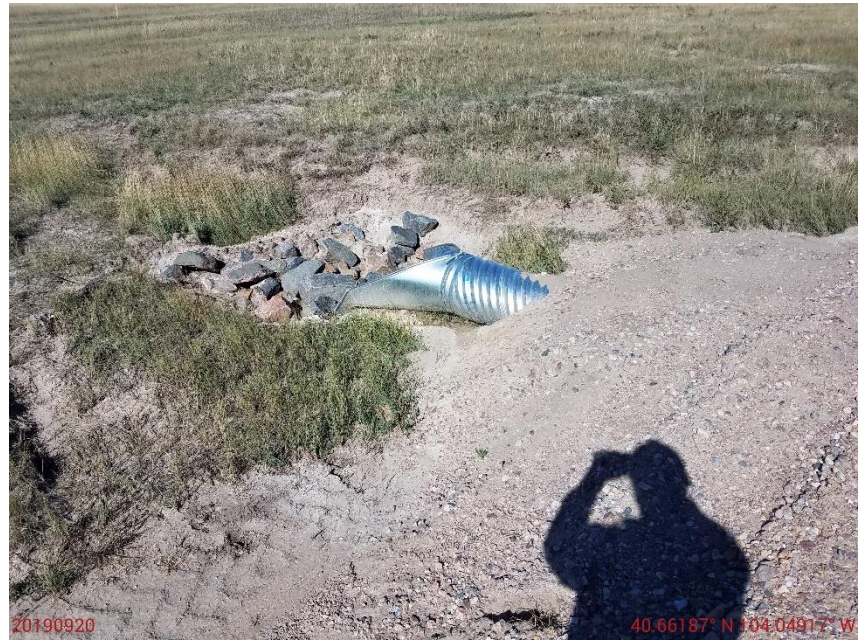
Photo 24: Photo taken from the culvert on the access road north of the pad. Photo shows sufficient outlet protection has not been installed above culvert outlet. Erosion degradation around culvert evident.
