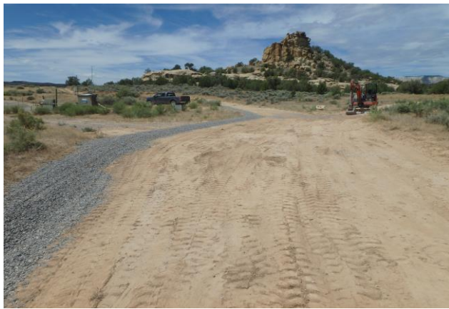
Bar Ditch / Earthen Berm Installed at Pad Entrance
