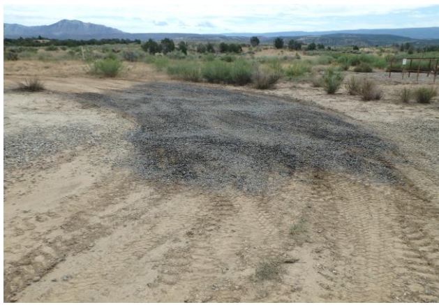
Ruts / Ponding Repaired on Access Road
