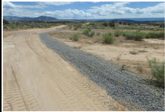
Bar Ditch / Earthen Berm Installed at Pad Entrance
