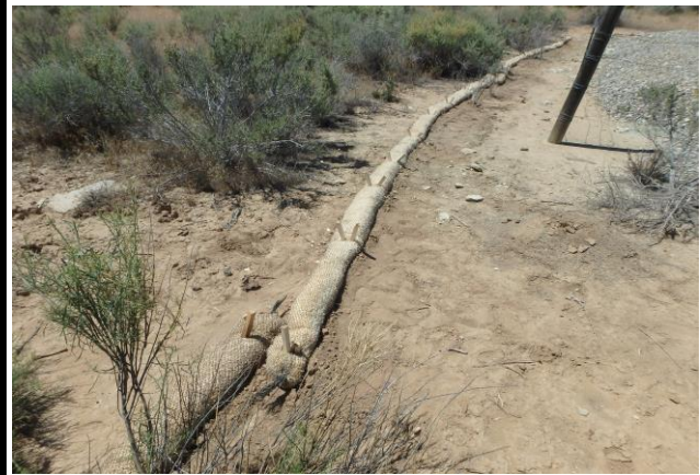
Excelsior Wattle Installed on South Side of Pad
