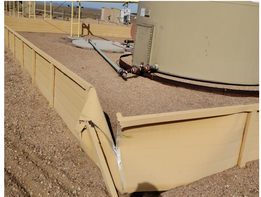
Photo #2 Picture taken from the SE corner, Berm wall is Mangled up.
