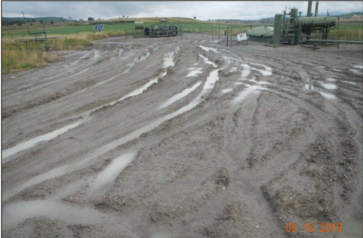
Photo 1. View of the project area from the well pad entrance facing center. Well pad is deeply rutted and water is ponding on working area. Stabilization measures are needed.
