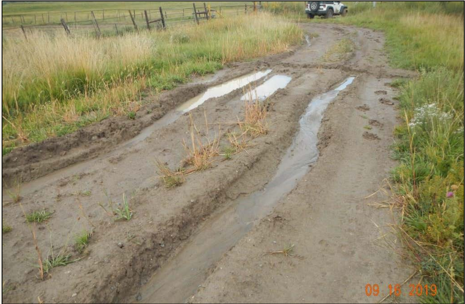
Photo 2. View of rutting up to 12 inches deep on the well pad access road.
