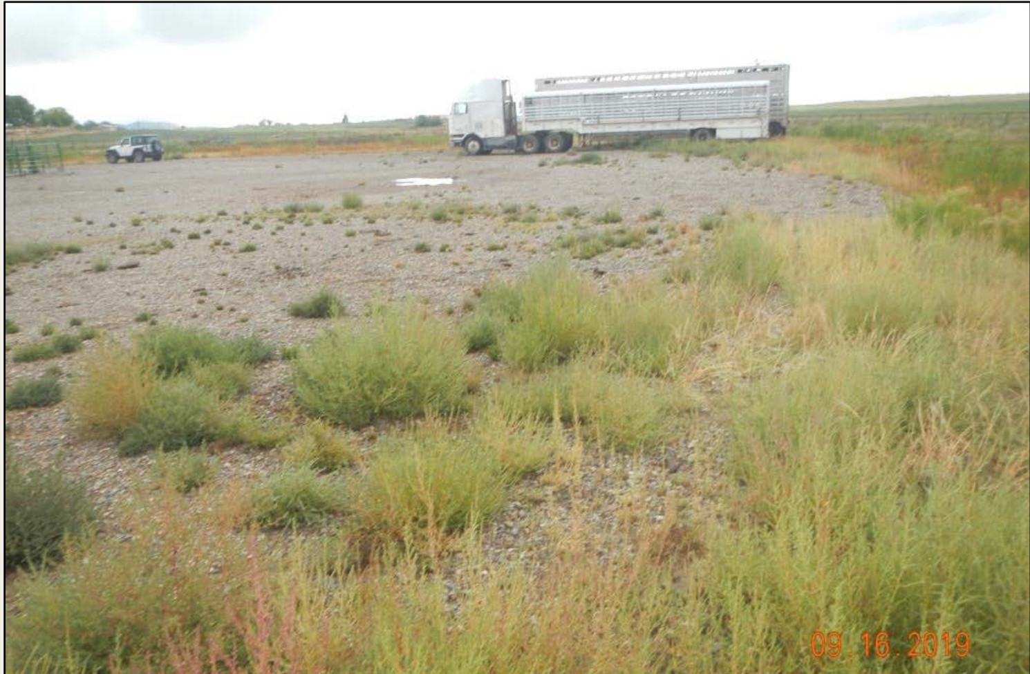
Photo 3. View of the southern project area from the western corner facing southeastward. Truck parked on well pad shows that portions of the southern project area are not needed for production operations and need reclamation.
