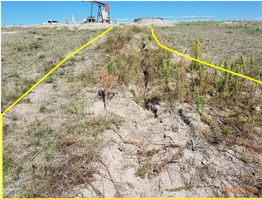
Photo 11: Photo taken from the adjacent lands south of the location, facing north. Photo shows erosion degradation and sediment deposition from stormwater runoff on the adjacent lands.
