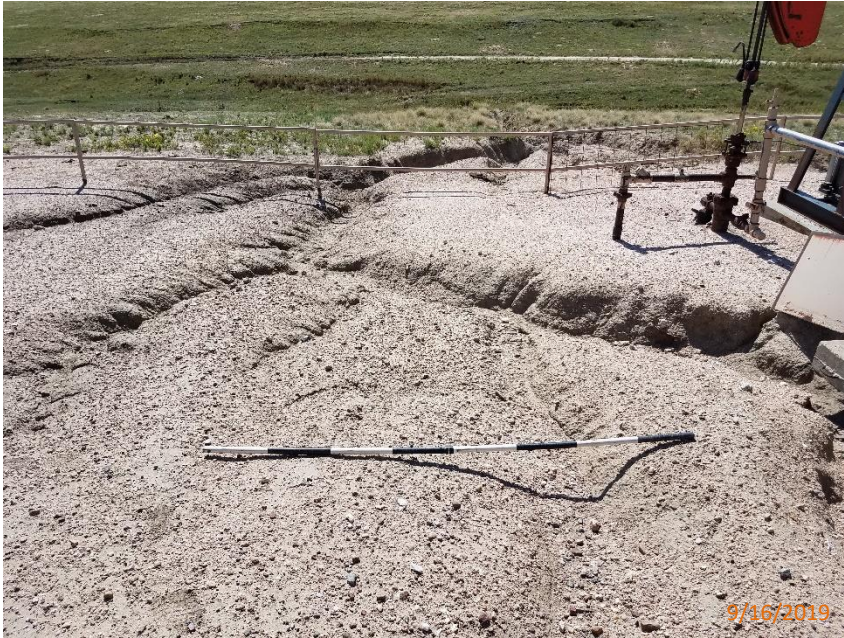
Photo 7: Photo taken from the location, facing south. Photo shows Stormwater erosion degradation is compromising the integrity and stability of the location. Additionally, photo shows stormwater runoff has also caused degradation to the adjacent lands below the location. Two meter (6.5 feet) metal pole for reference
