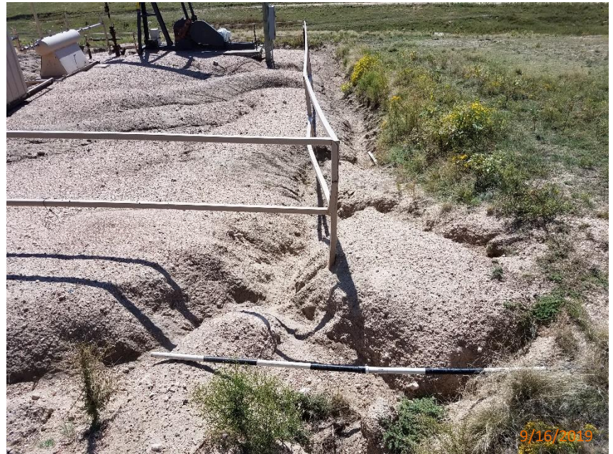
Photo 2: Photo taken from the northwest corner of the location, facing south. Photo shows stormwater erosion degradation. Two meter (6.5 feet) robel pole for reference
