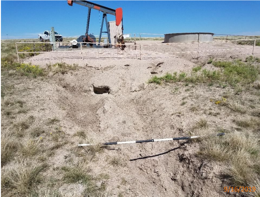
Photo 9: Photo taken from the adjacent lands south of the location, facing north. Photo shows stormwater runoff from the location has caused degradation to the adjacent lands.
