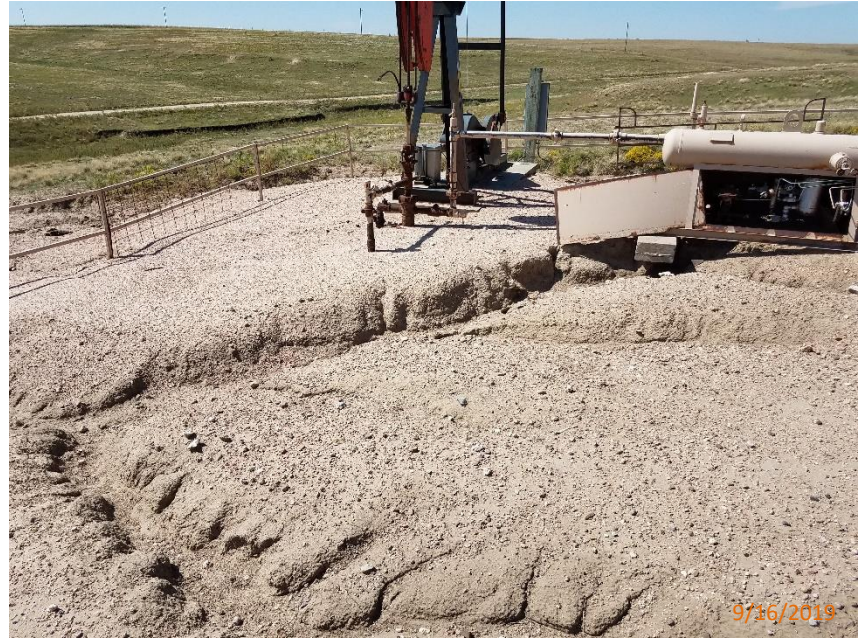
Photo 6: Photo taken from the location, facing west. Photo shows stormwater erosion degradation. Operator has failed to conduct sufficient stormwater management in accordance with 1002.f. Stormwater erosion is compromising the stability of the location.
