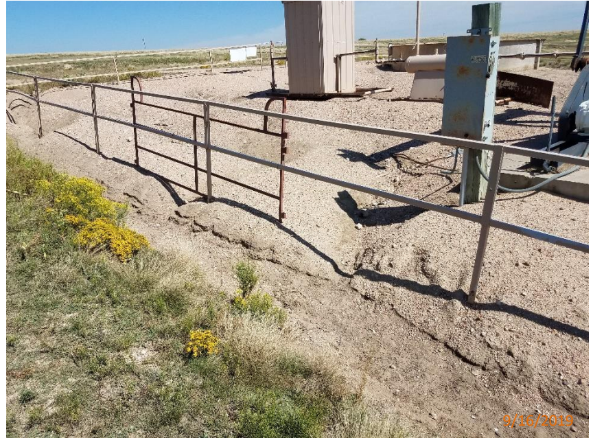
Photo 8: Photo taken from the west end of the location, facing north east. Photo shows stormwater erosion degradation on location. Photo also shows erosion degradation to the adjacent lands due to stormwater runoff from the location.
