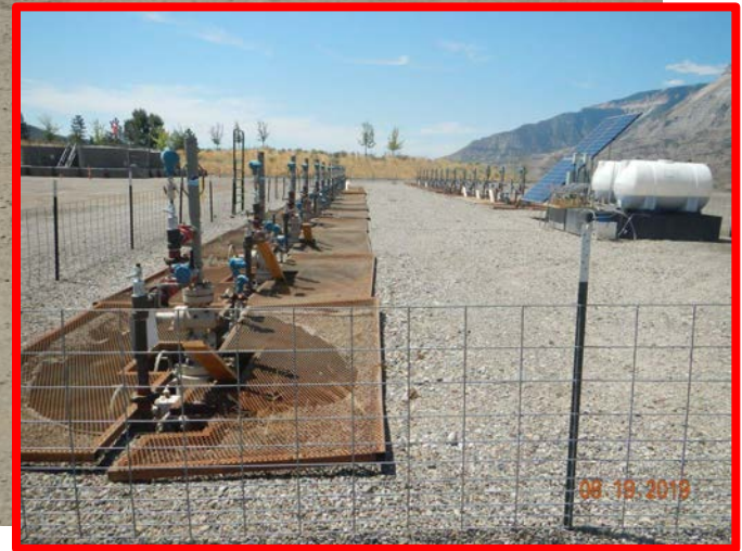
Photo#1: Overview of Location to Southwest. Wildlife escape boards have been installed.
