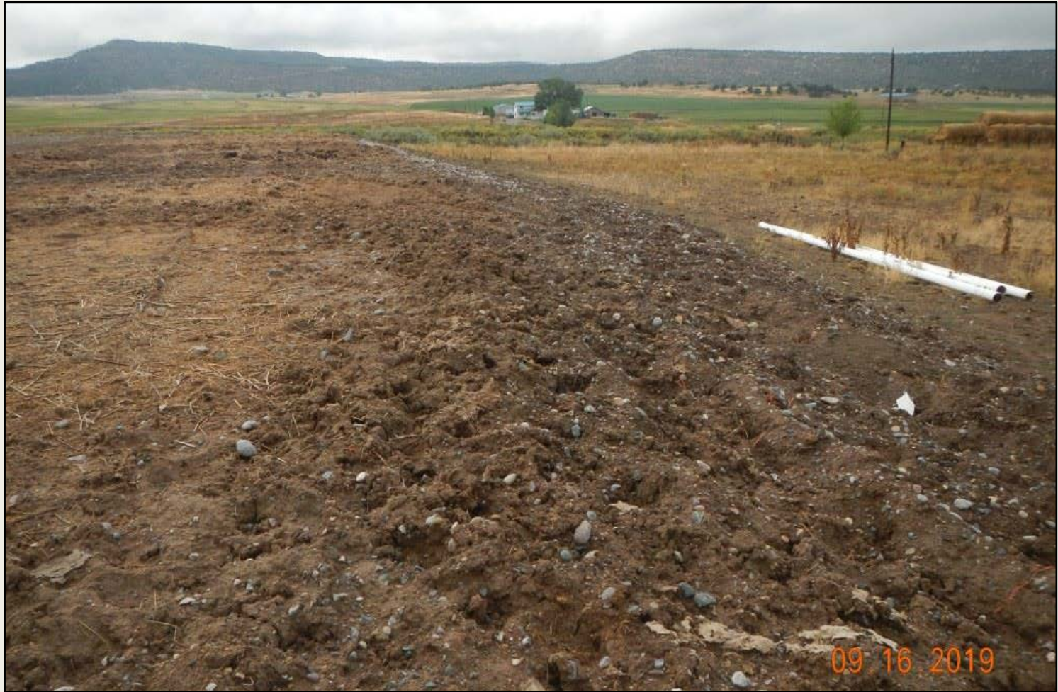
Photo 2. View of the western fill slope facing southward. Little vegetation present here. Revegetation is needed.
