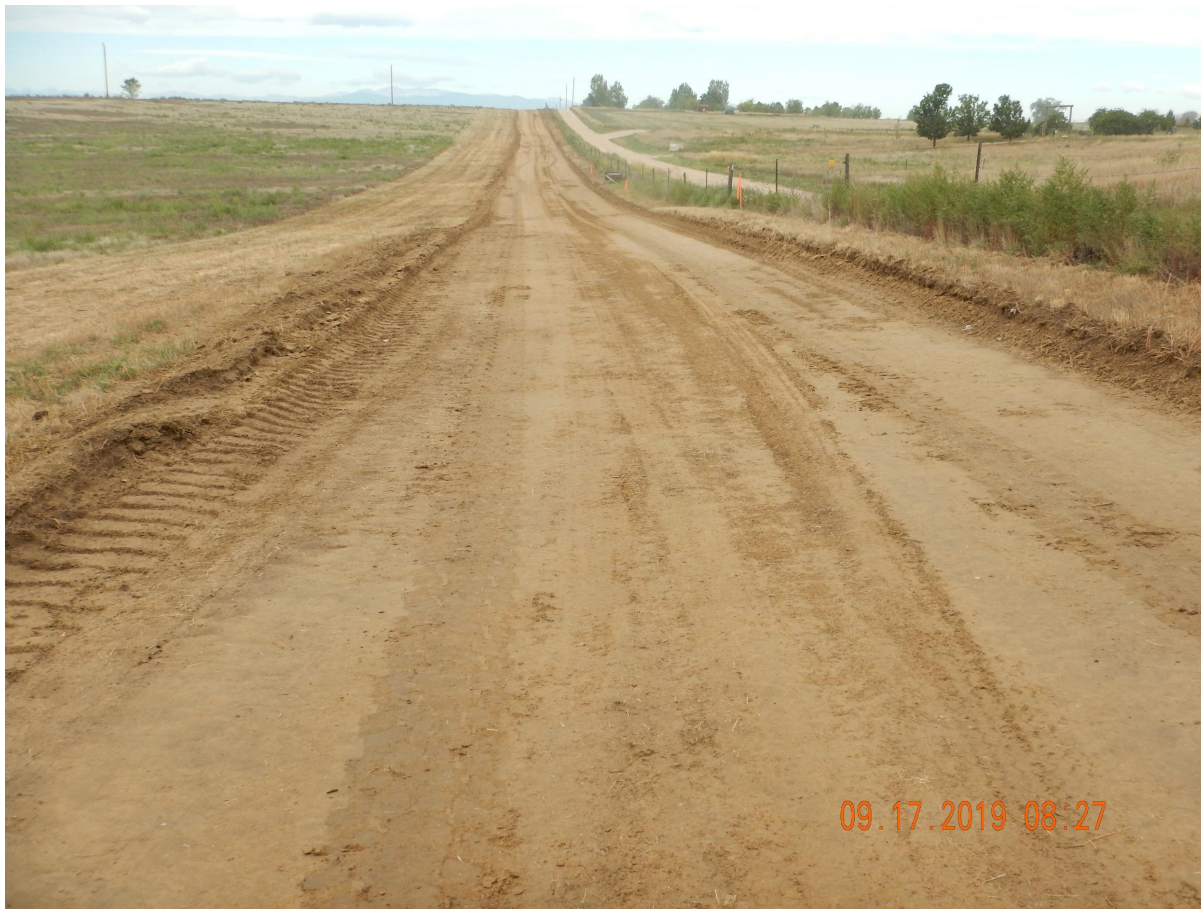
Photo 1. Photo taken from the eastern portion of the access road, facing West. Photo illustrates the Operator has salvaged some topsoil along the access road and has stored it at the location.
