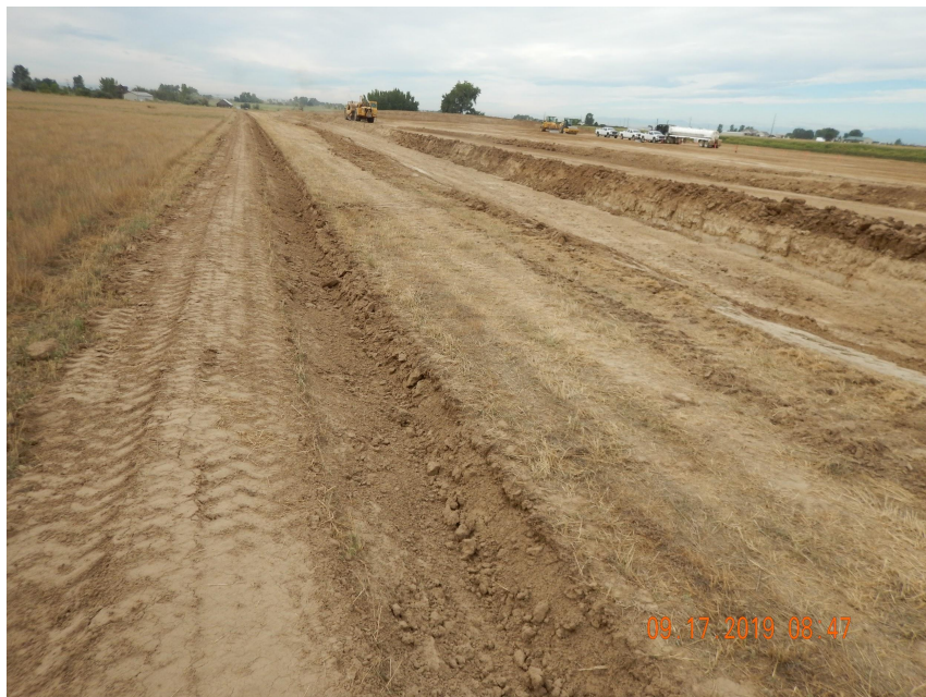
Photo 2. Photo taken from the eastern perimeter of the location, facing South. Photo illustrates a ditch and berm BMP which has been installed around the entire perimeter of the location.
