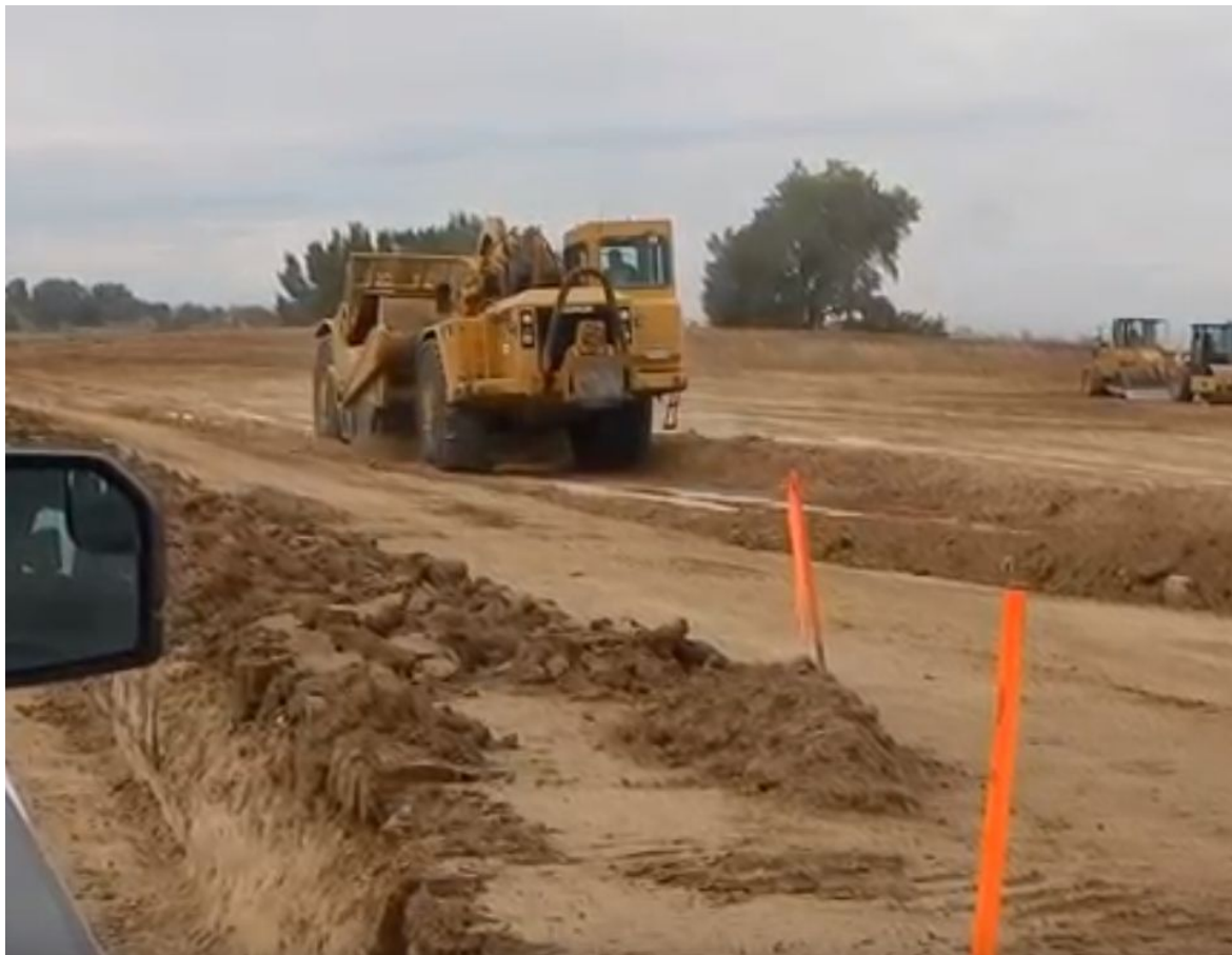
Photo 8. Photo taken from the northeastern location, facing South. Photo is illustrating the Operator scraping topsoil which was placed on the eastern production pad as fill material. Photo 9 illustrates topsoil that was placed on the eastern production pad as fill material.
