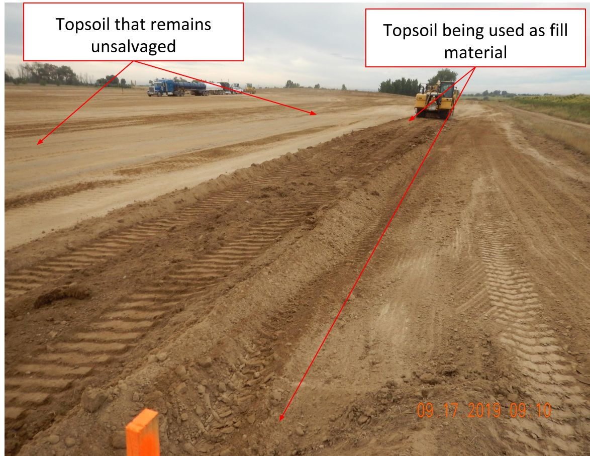
Photo 10. Photo taken from the northwestern well pad location, facing South. Photo illustrates the Operator placing topsoil on the northwestern well pad as fill material. Photo also illustrates topsoil that remains unsalvaged from the well pad.
