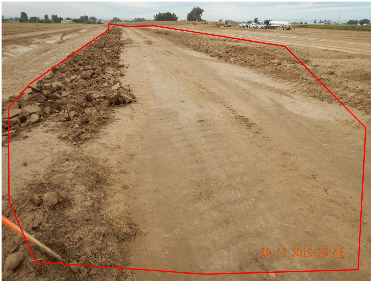
Photo 7. Photo taken from the northeastern location, facing South. Photo is illustrating topsoil (all within the red line) that was scraped by the Operator and used as fill material on the eastern production pad. Photo 8 illustrates the scraping operation.
