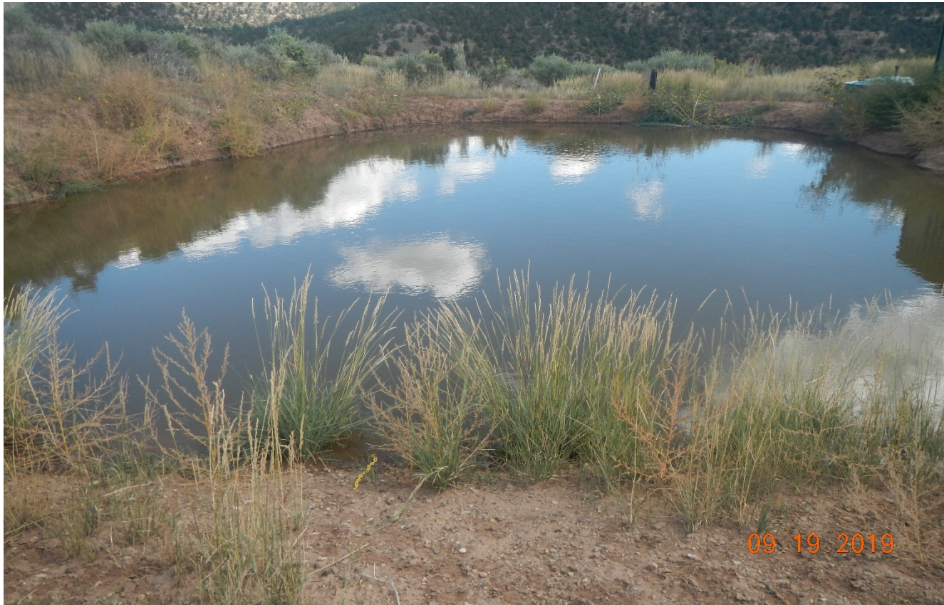
Photo 2. Water level at pit is at 2ft freeboard and needs to be lowered.
