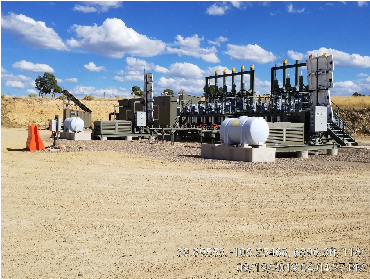
Photo 2. Separator, RTU, chemical, and header.
