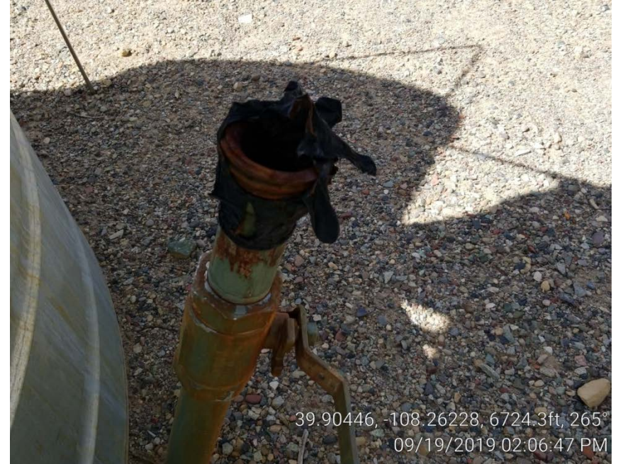
Photo 4. Riser capped with glove.
