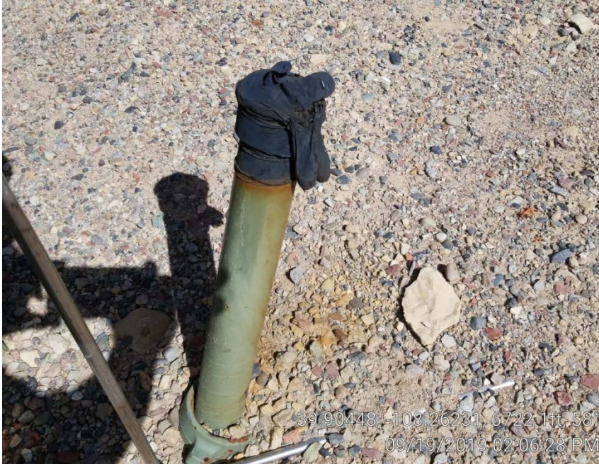
Photo 3. Riser capped with glove.
