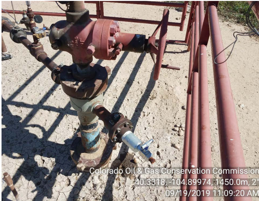
Master valve and stained soil on Gold 9A-DU
