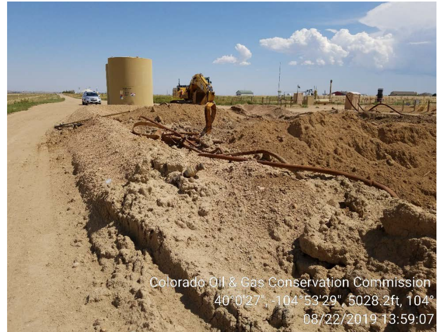
Photo 6 Open excavation. Note pipes removed from excavation .
