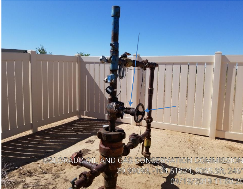
Pic 11 venting wellhead equipment
