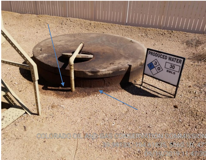
Pic 9 Produced water vault/leak/spill
