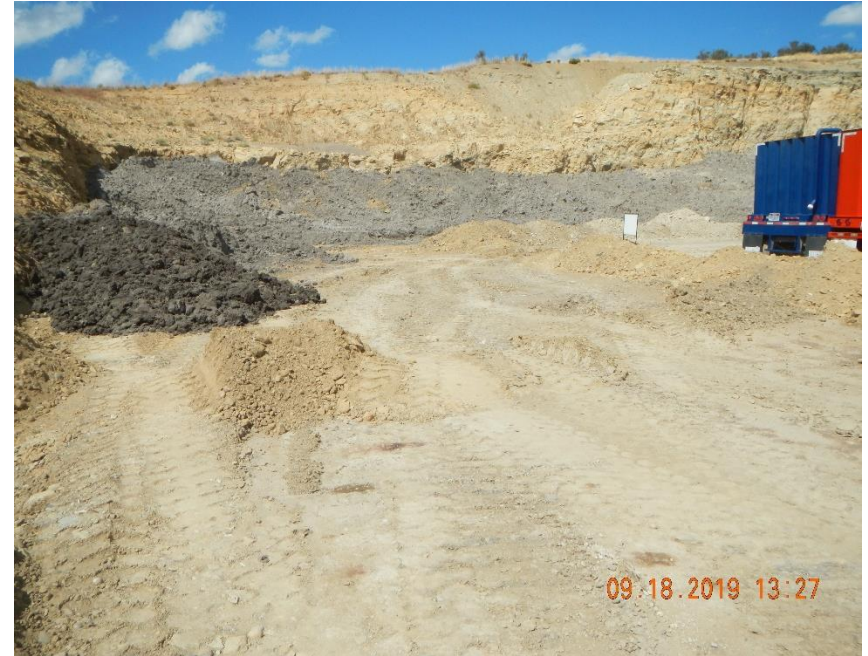
Uncompleted and uncompacted berm where cutting are being brought in.
