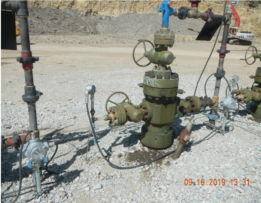
Stained ground surfaces at and around wells.
