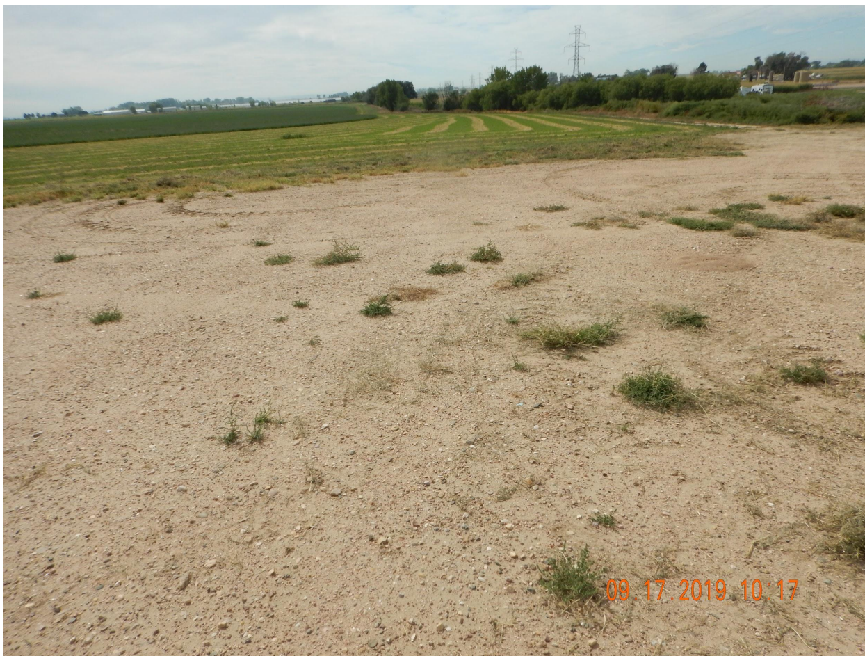
Photo 2. Photo taken from the battery location, facing South. Photo illustrates the Operator has failed to complete final reclamation activities. Note: Surface owner was at the tank battery location and indicated the desire to leave the gravel in-place for hay and equipment storage.
