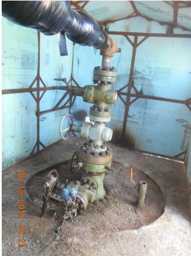
Injection wellhead inside housing
