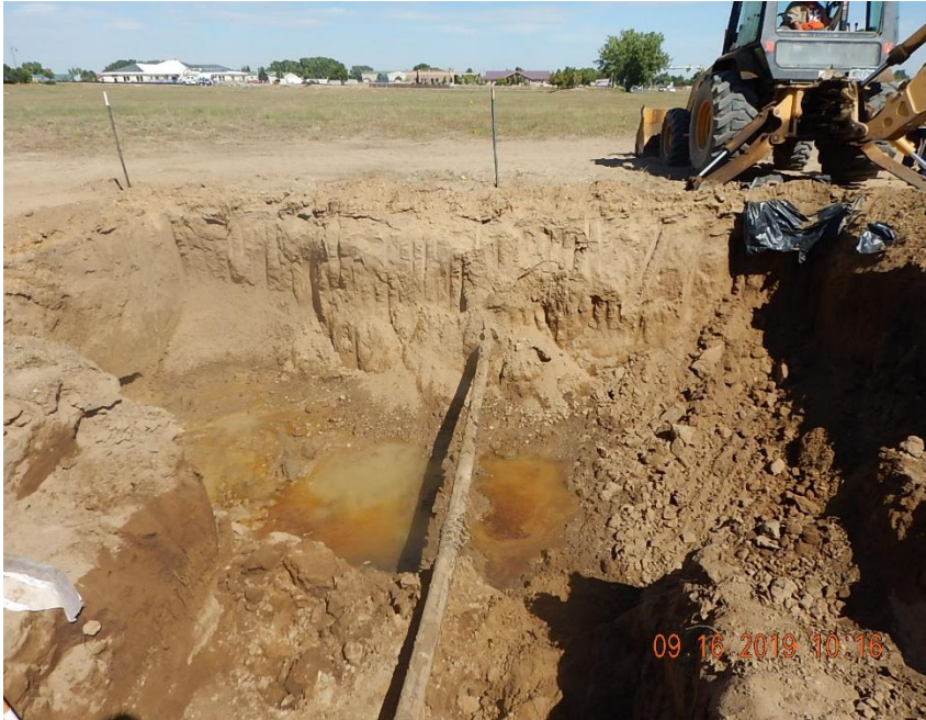
View of the excavation and 4" Carbon Steel crude oil consolidation flowline exposed in excavation. Impacts to ground water can be seen. (view to North)
