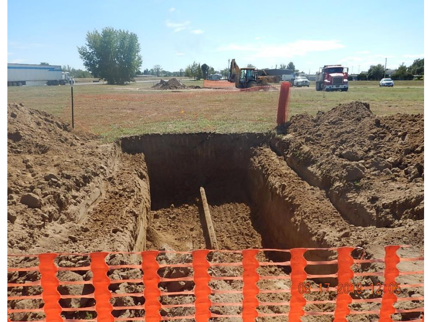
View from the excavation completed to expose the crude oil consolidation line for the repair to the south excavation where the spill occurred.
