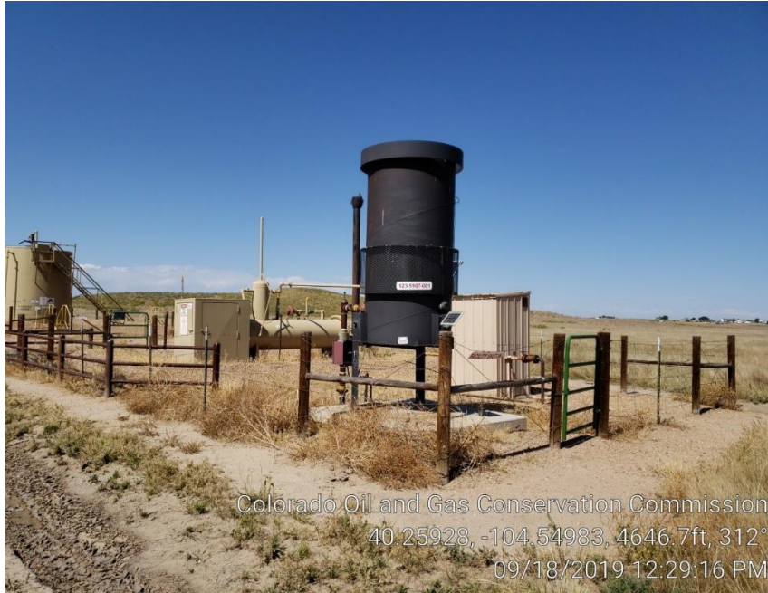
Photo #1 Separator, ECD, Meter Run & Weeds
