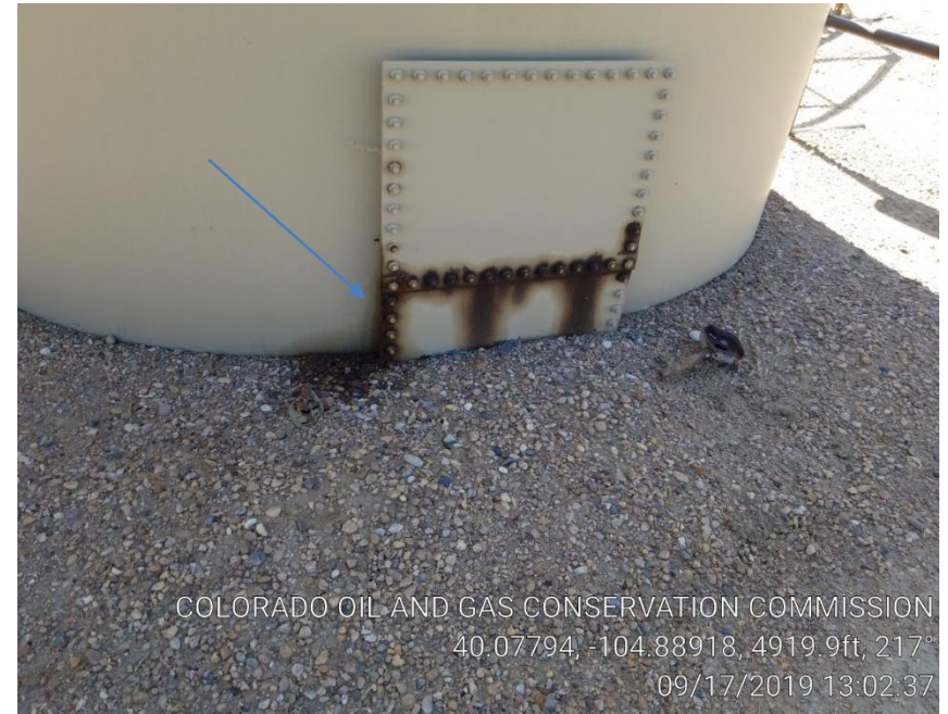
Pic 10 mechanical conditions/stained soil
