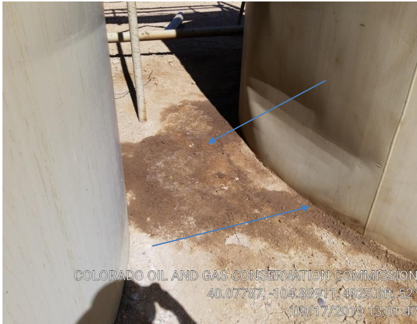
Pic 5 stained soil/possible leak on bottom of tank
