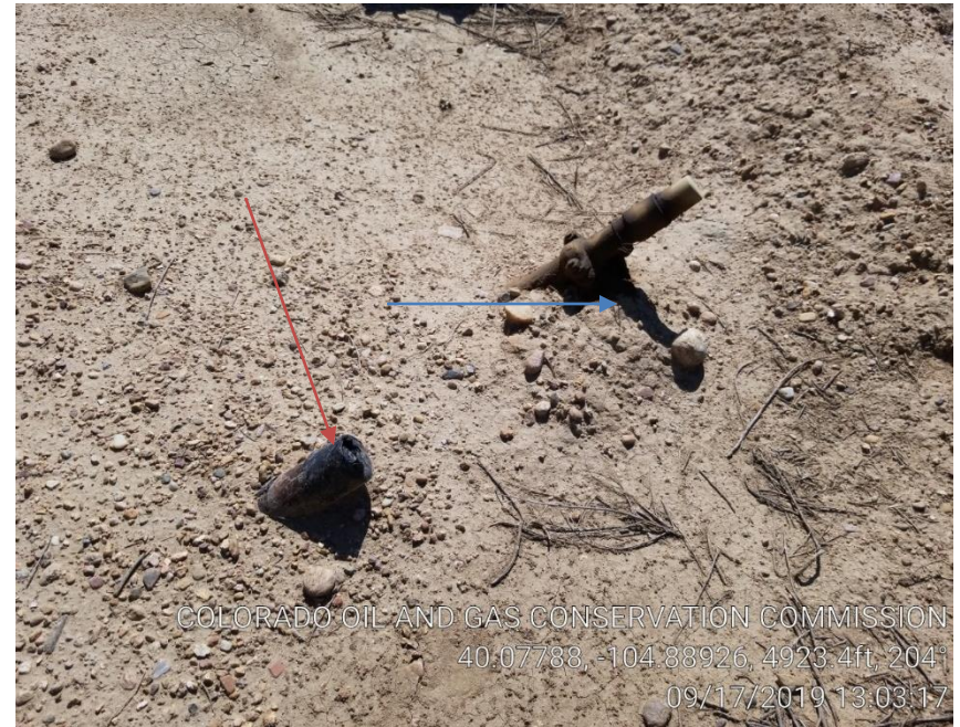
Pic 12 unused not LOTO riser/stained soil
