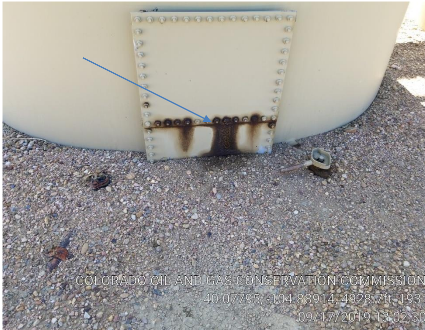
Pic 9 mechanical conditions/stained soil
