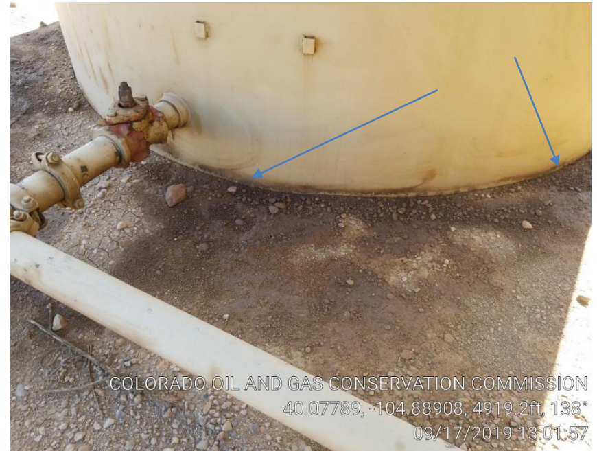
Pic 6 stained soil/possible leak on bottom of tank
