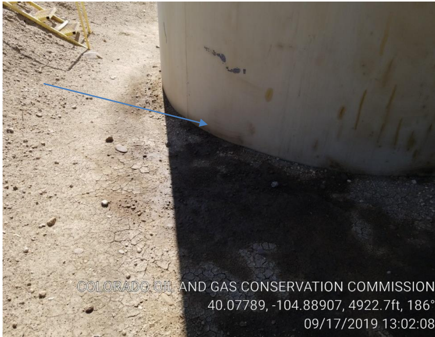
Pic 7 stained soil/possible leak on bottom of tank
