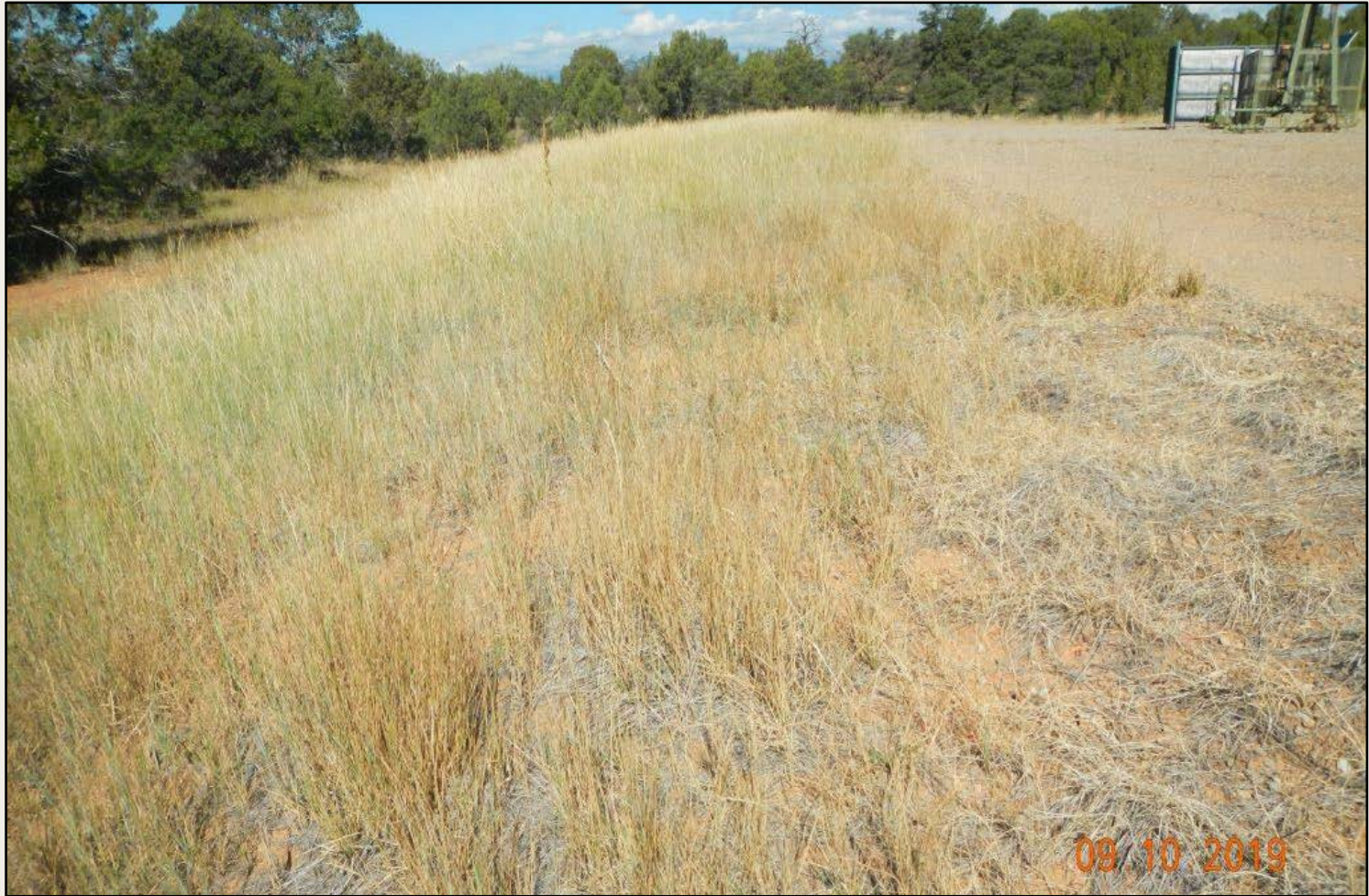
Photo 2. View of the southern fill slope from the southeastern edge facing westward. Revegetation is progressing with western wheatgrass and intermediate wheatgrass.
