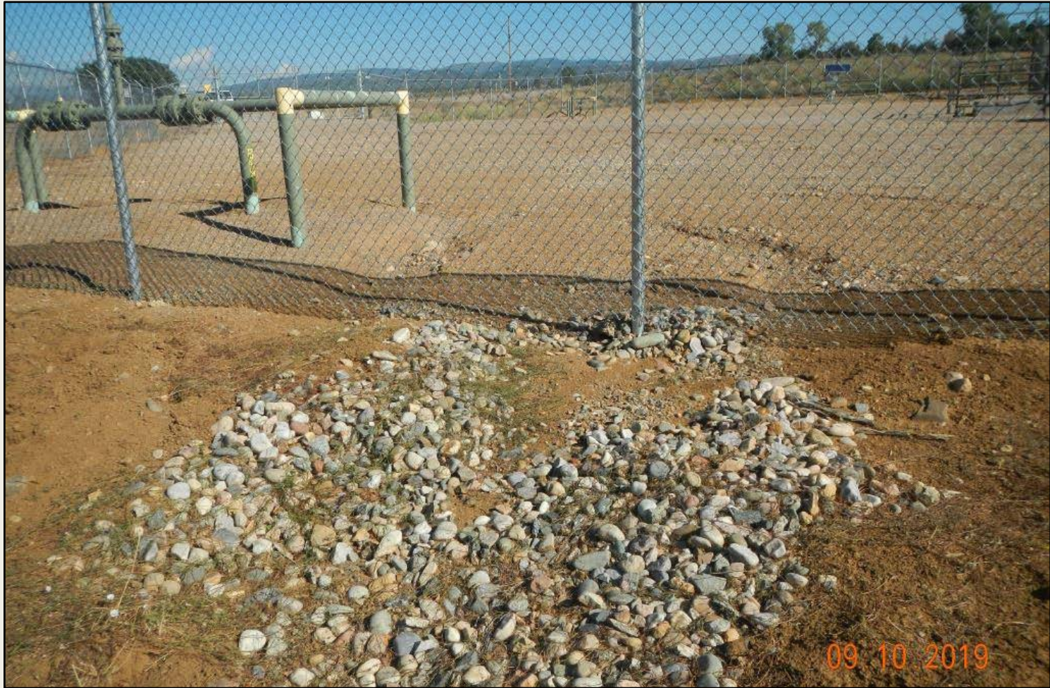
Photo 5. View of area where concentrated stormwater flows off of the southern project area. This stormwater BMP is not adequate here as bare soils throughout the revegetation area are not stabilized.
