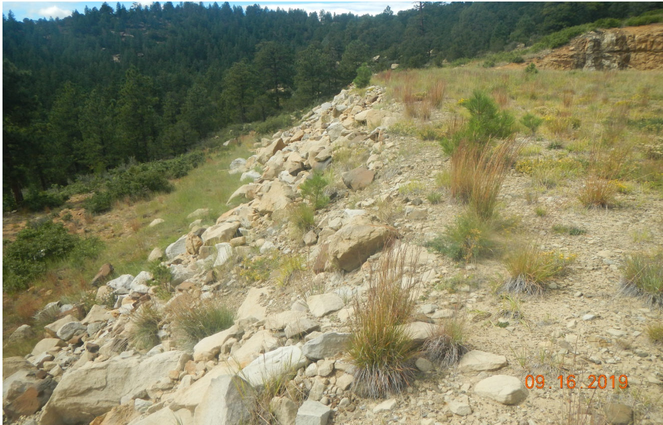
Photo 7. Facing west toward the fill slope which is mostly rock.
