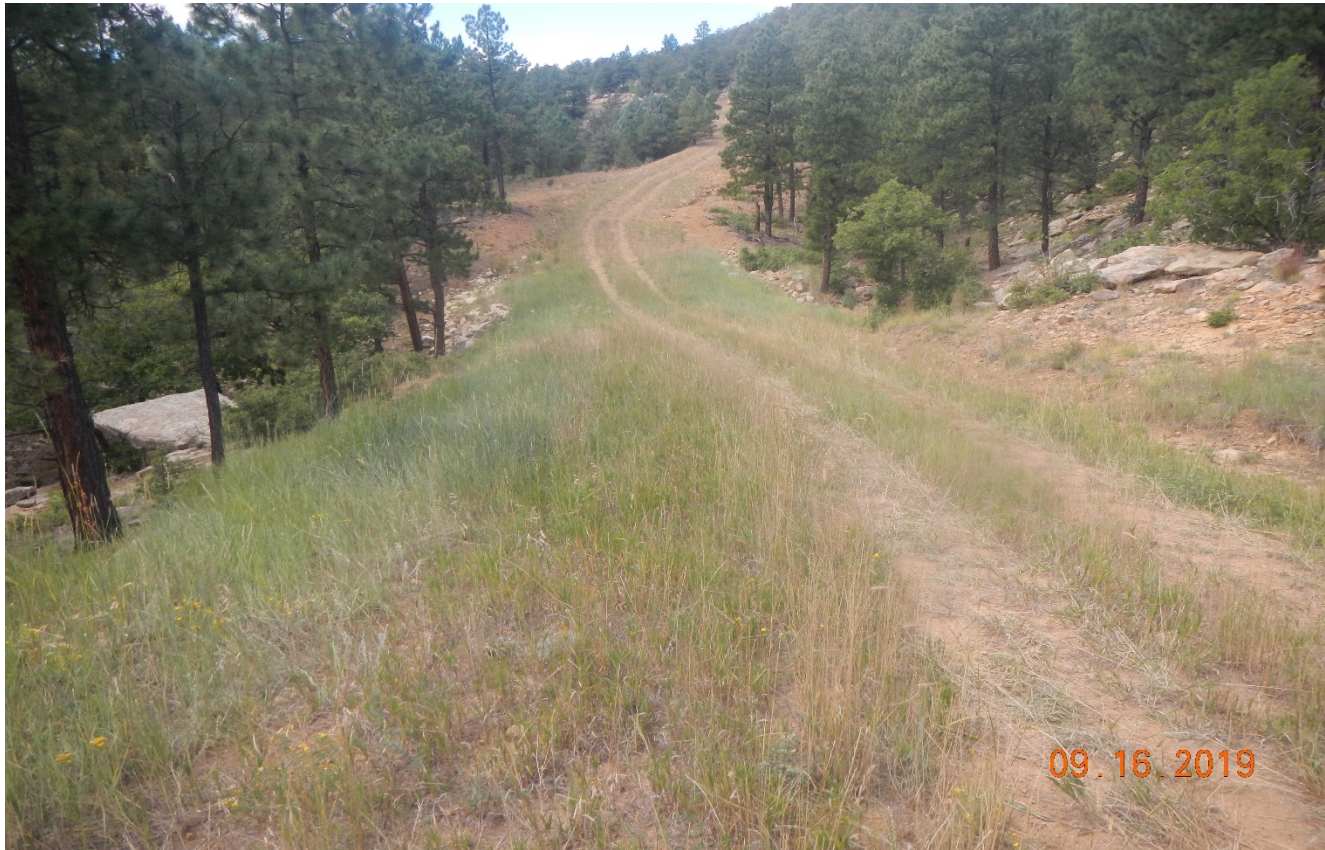
Photo 1. Facing northwest along the access road.
