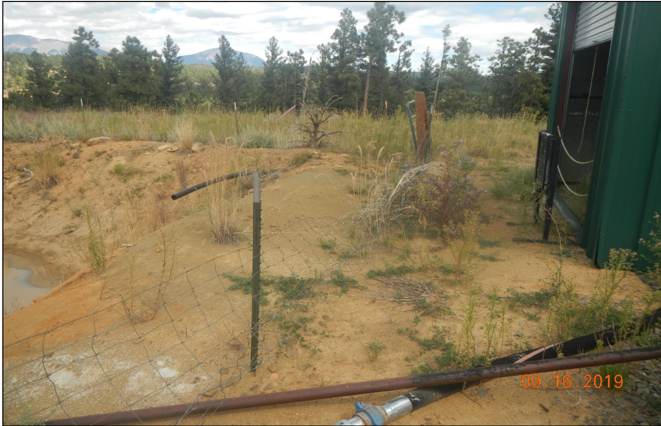
Photo 5. The fence is not maintained around the pit.
