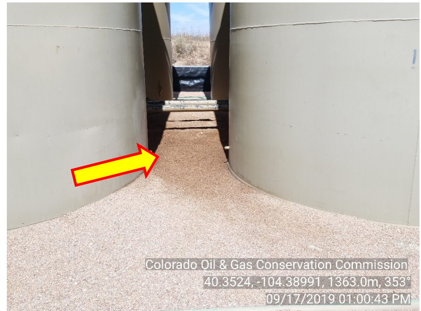
Photo #6 North Platte 14-36, X-D-35HZ Battery Latham F-J-35HZ Stained soil Crude oil tanks 2, 3
