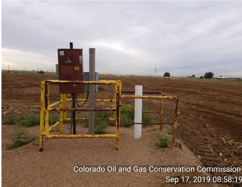
Photo 3 electric breaker box for PU is in the Off position.
