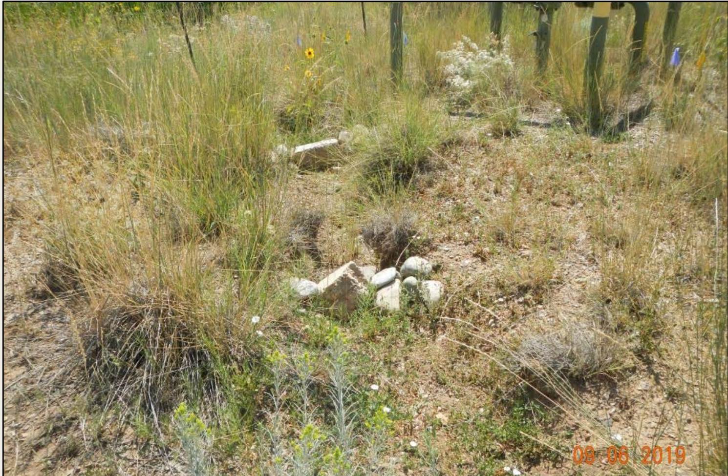
Photo 2. View of rock checks in the southern project area. These are not a sufficient stormwater BMP for this area.
