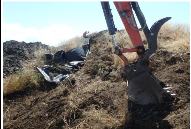
Installing Silt Fence around Upper Topsoil Pile
