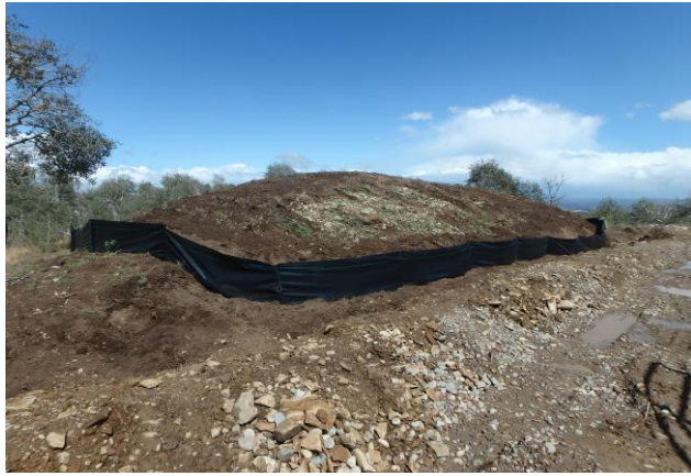
Silt Fence around Northeast Topsoil Pile
