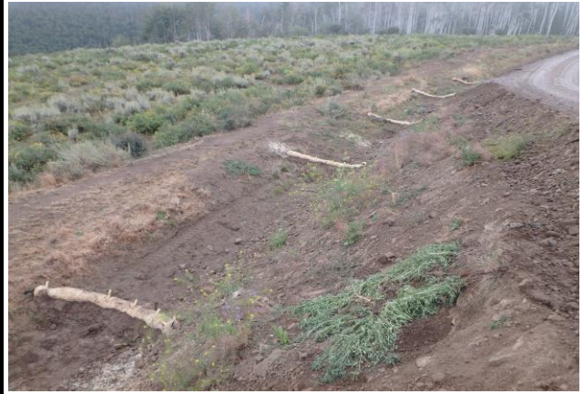
Wattle Checks Installed along Access Road
