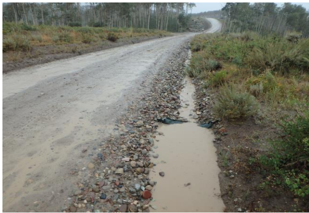
Rock Sock Working along Access Road
