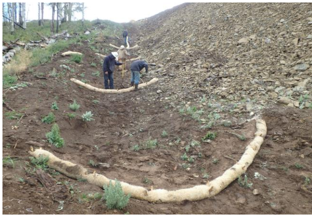
Installing Wattle in Channel on North Side of Pad
