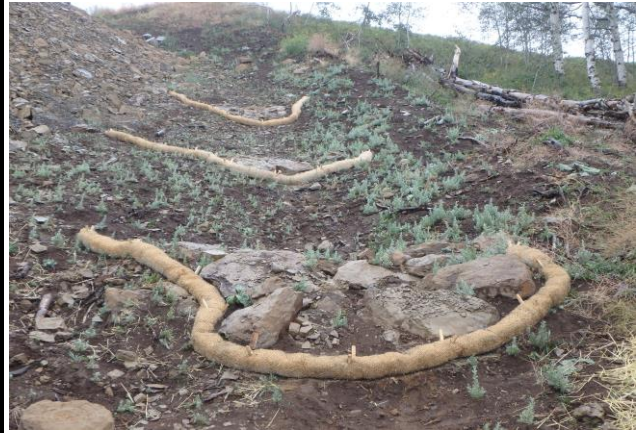
Wattle Installed below Existing Rock Checks
