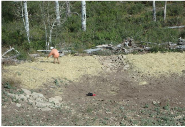
Hand Crimping Mulch on North Outlet
