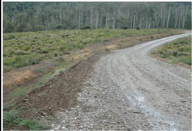
Berm Installed along Access Road
