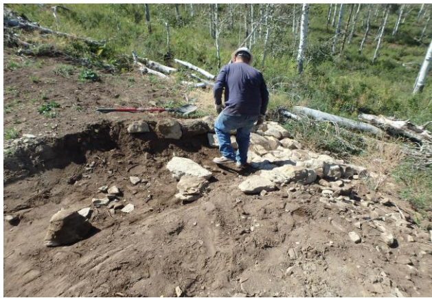
Installing New Rock Apron on CC 604-41-32 Pad
