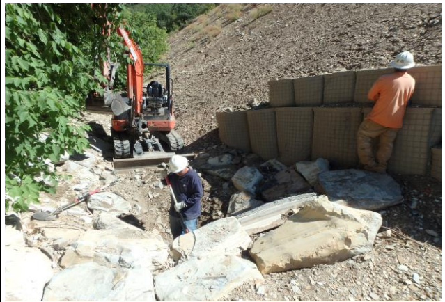
Removing Large Rocks in Culvert on CC 697-16D
