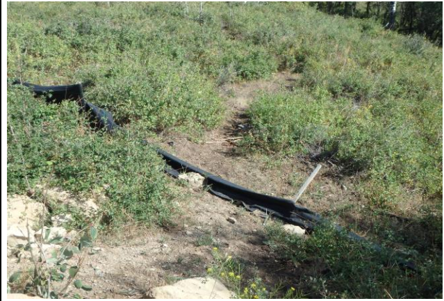
Silt Fence Damaged at Cattle Trail Crossing
