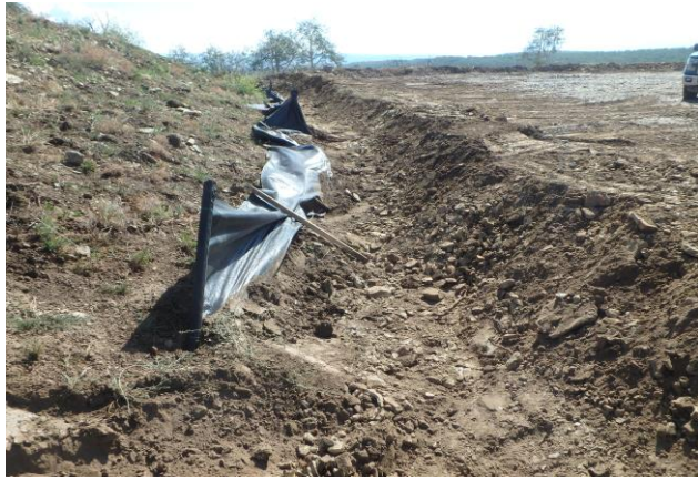
Silt Fence Damaged while Installing Earthen Berm
