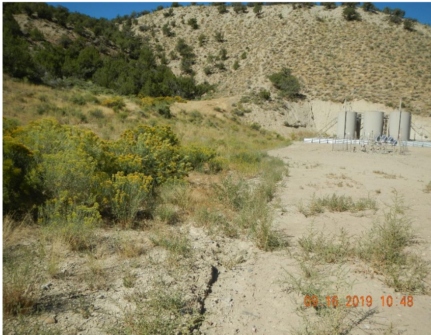
Sediment build up in ditch.
