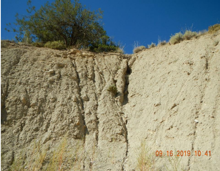
Cut wall behind tank battery is rilling and eroding in corner.
