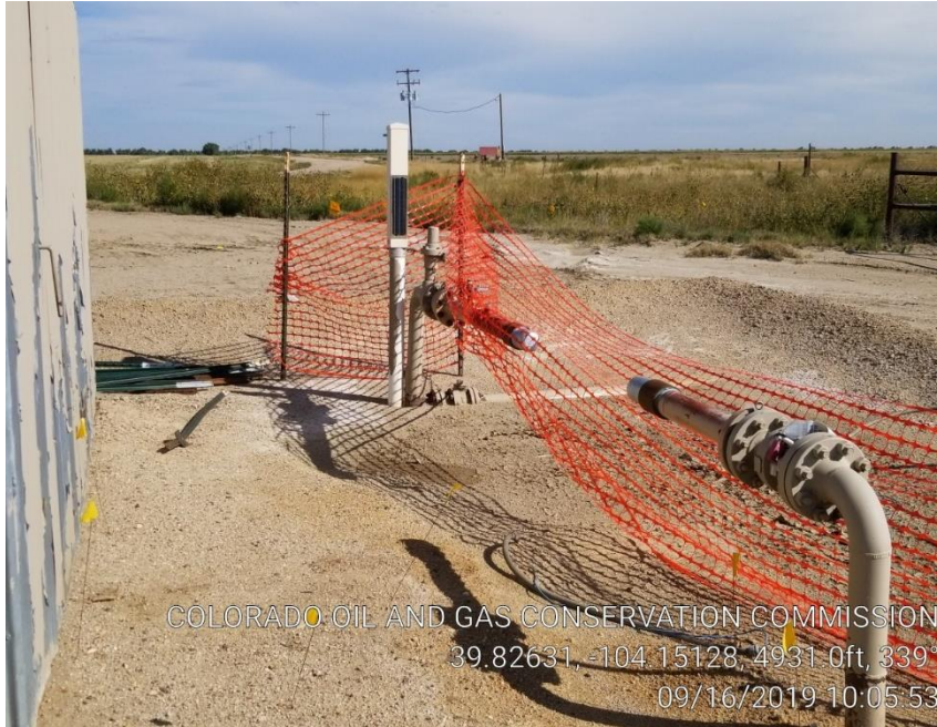
Pic 7 Midstream equipment de-commissioned
