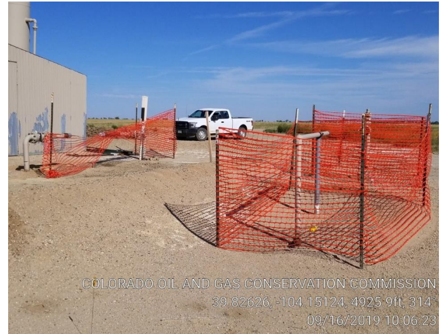
Pic 10 Midstream equipment de-commissioned
