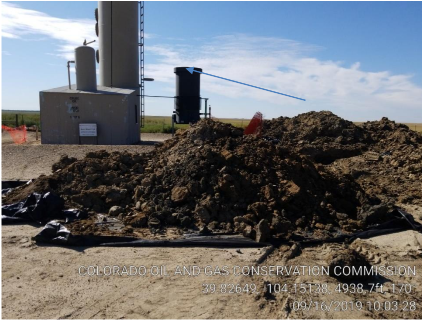
Pic 15 ECD, and vertical separator.
