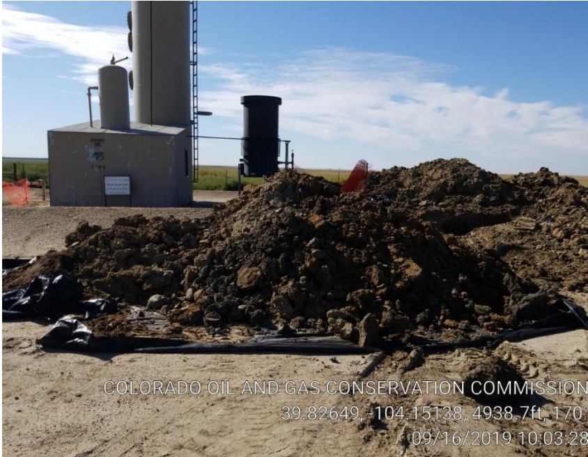
Pic 1 excavation of spill site
