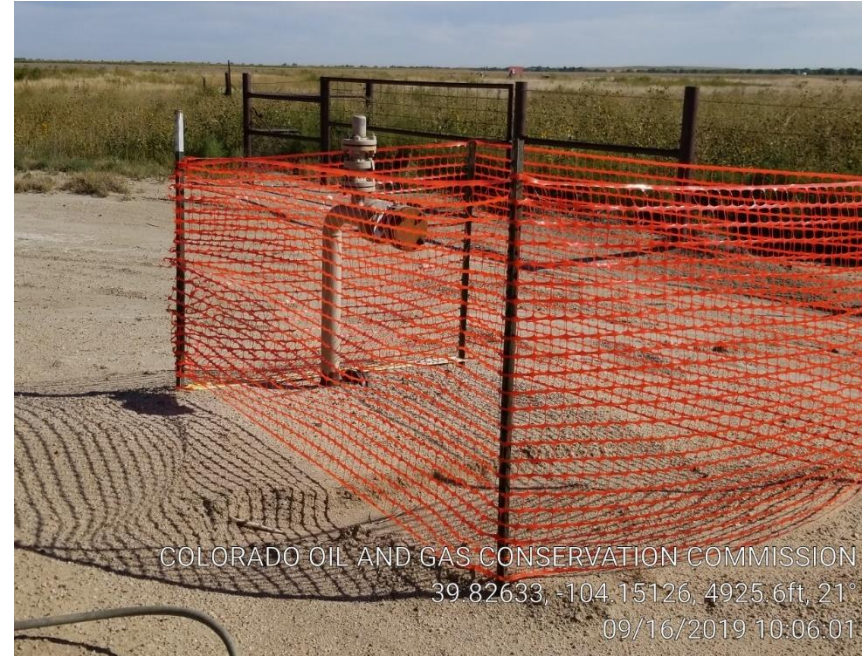
Pic 8 Midstream equipment de-commissioned
