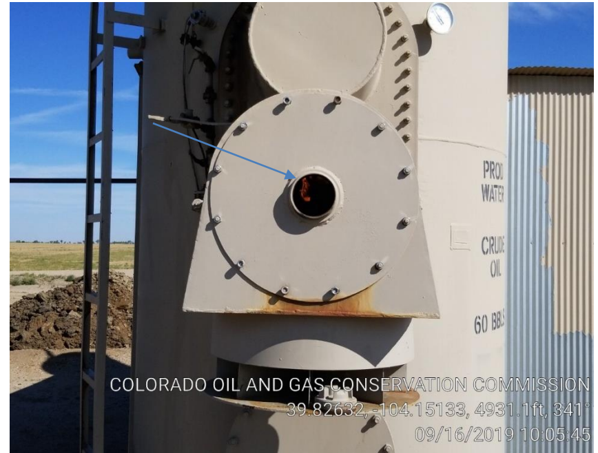
Pic 6 no cover on Vertical Heated Separator flange
