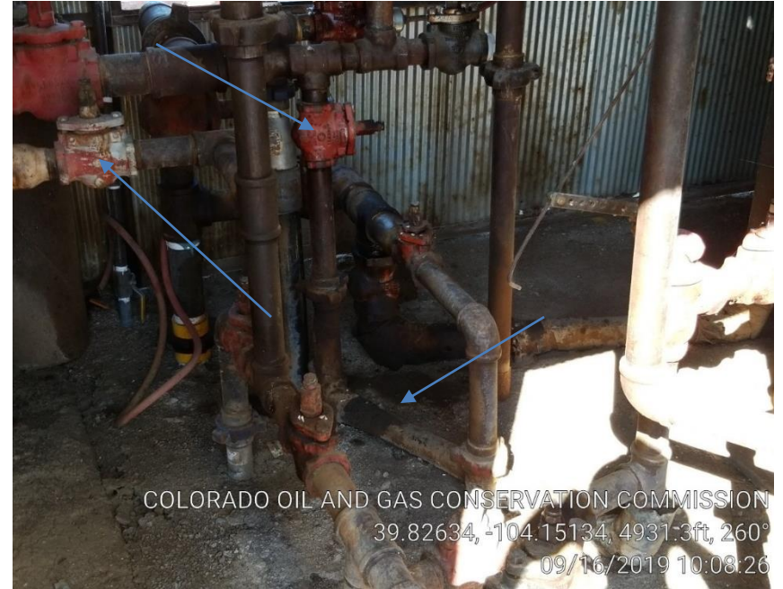
Pic 14 mechanical conditions/stained soil in separator house
