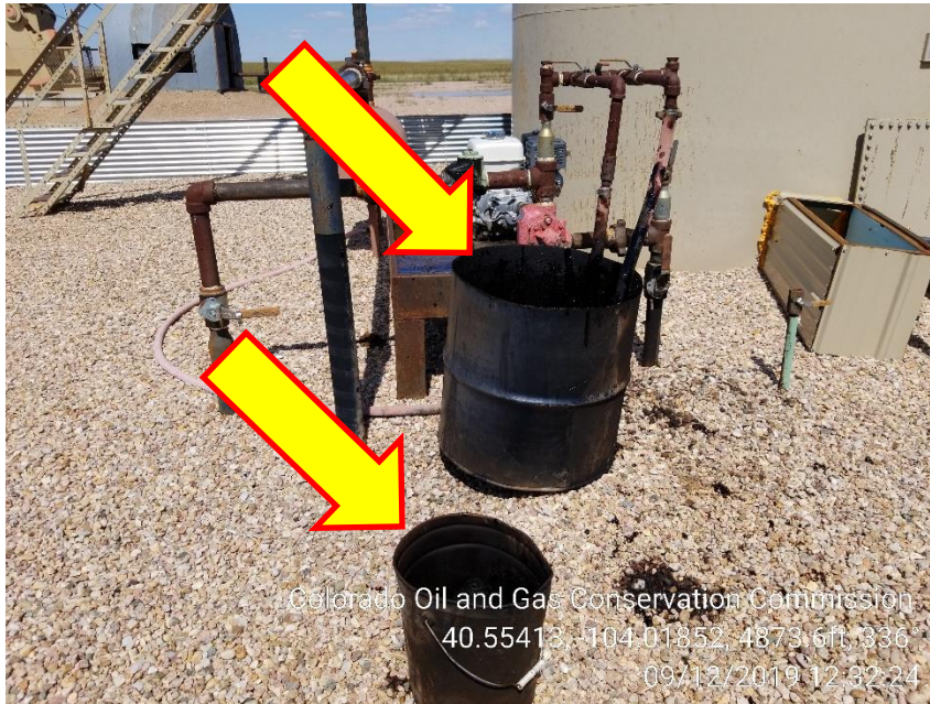
Photo 7 – Oily Wates at Recycle pump
