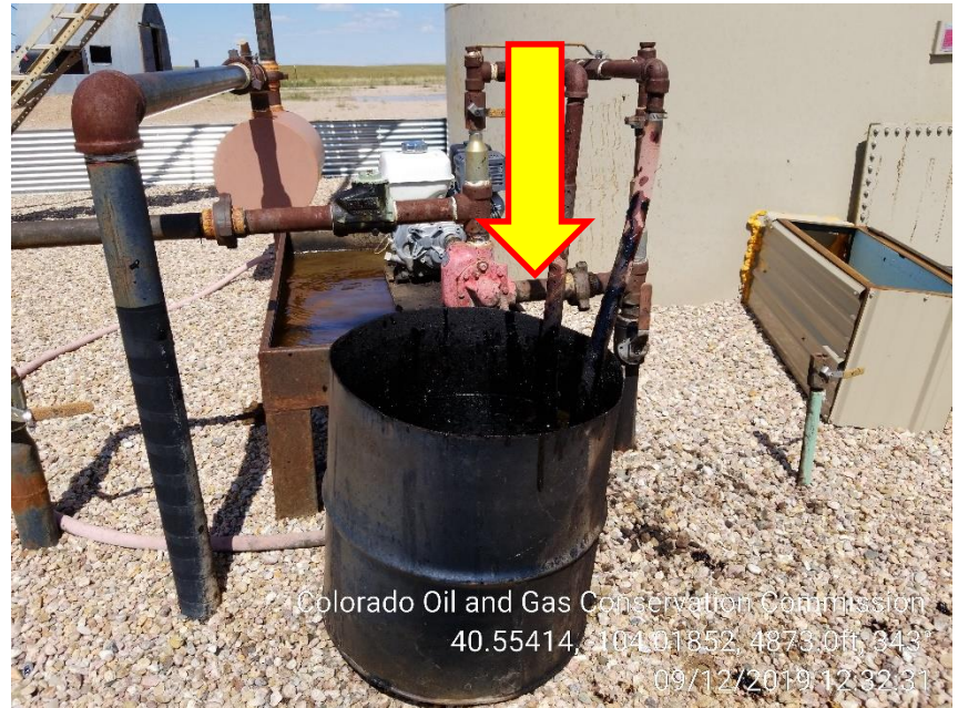
Photo 8 – Oily Wates at Recycle pump, dispose of and install Wildlife Netting
