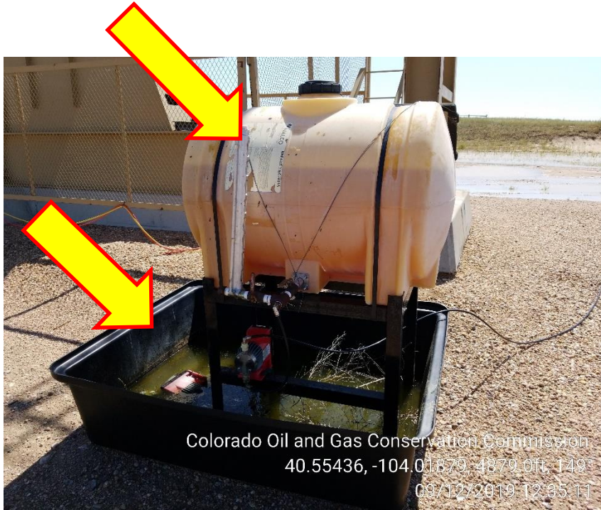
Photo 9 – Chemical Tank/Pump at Wellhead, Please install Wildlife netting. Label is fading, please consider new label.
