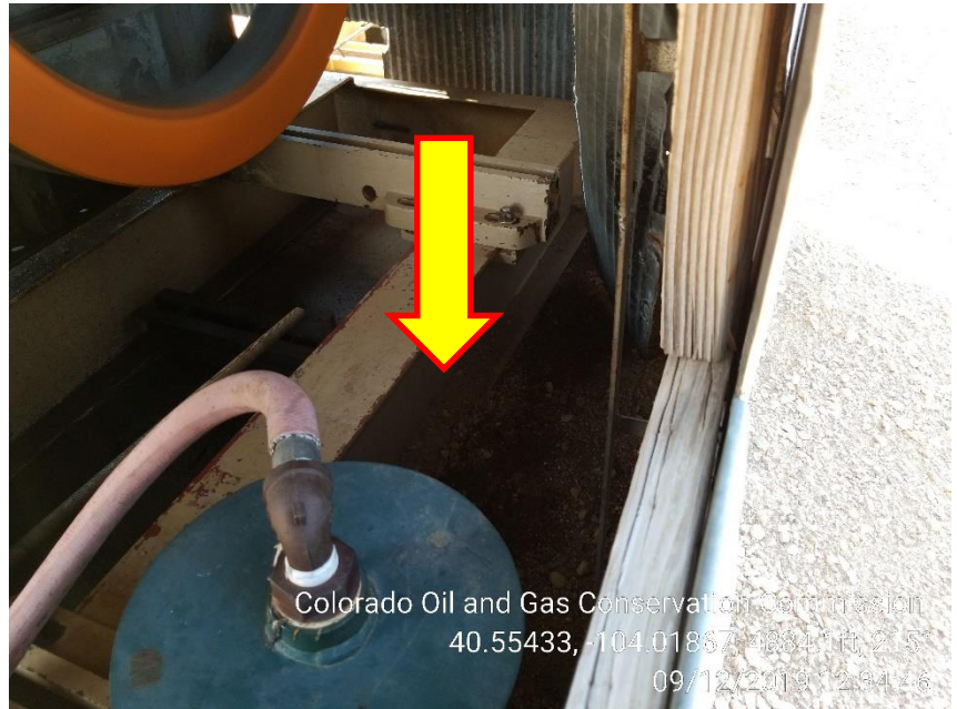
Photo 6 – Stained Soil at Engine Base
