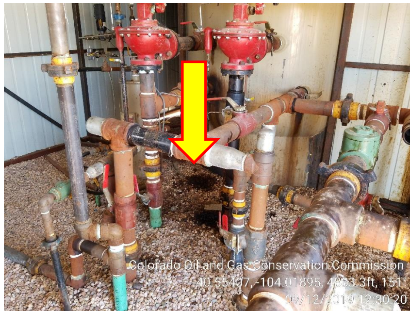
Photo 4 – Stained Soil inside Treater Shed
