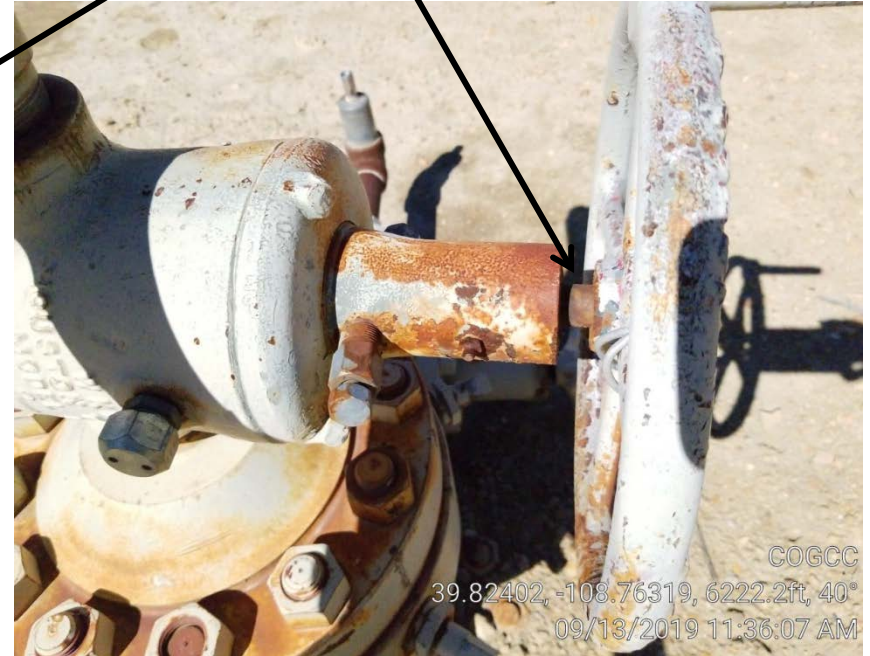
Photo 3. Well head master valve.
