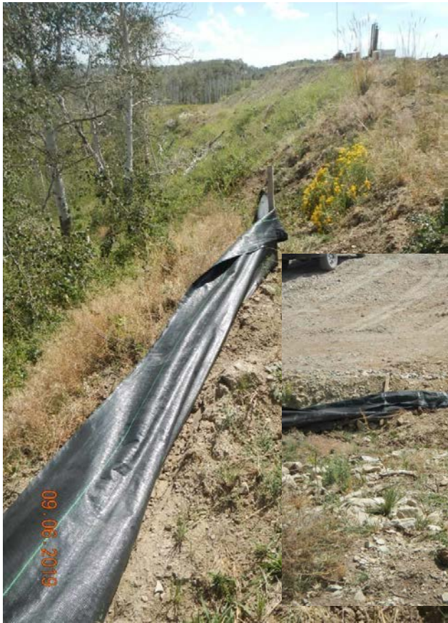
Photo#4: Silt fence is in disrepair.
