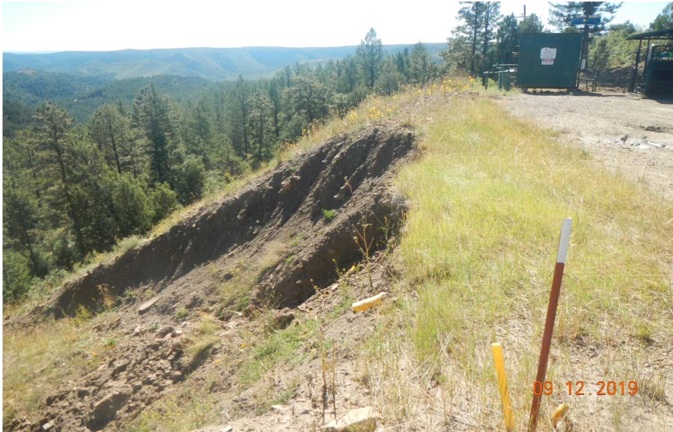
Photo 2. There is soil sloughing that occurred at the east side of the location. Corrective action of previous inspection not performed.
