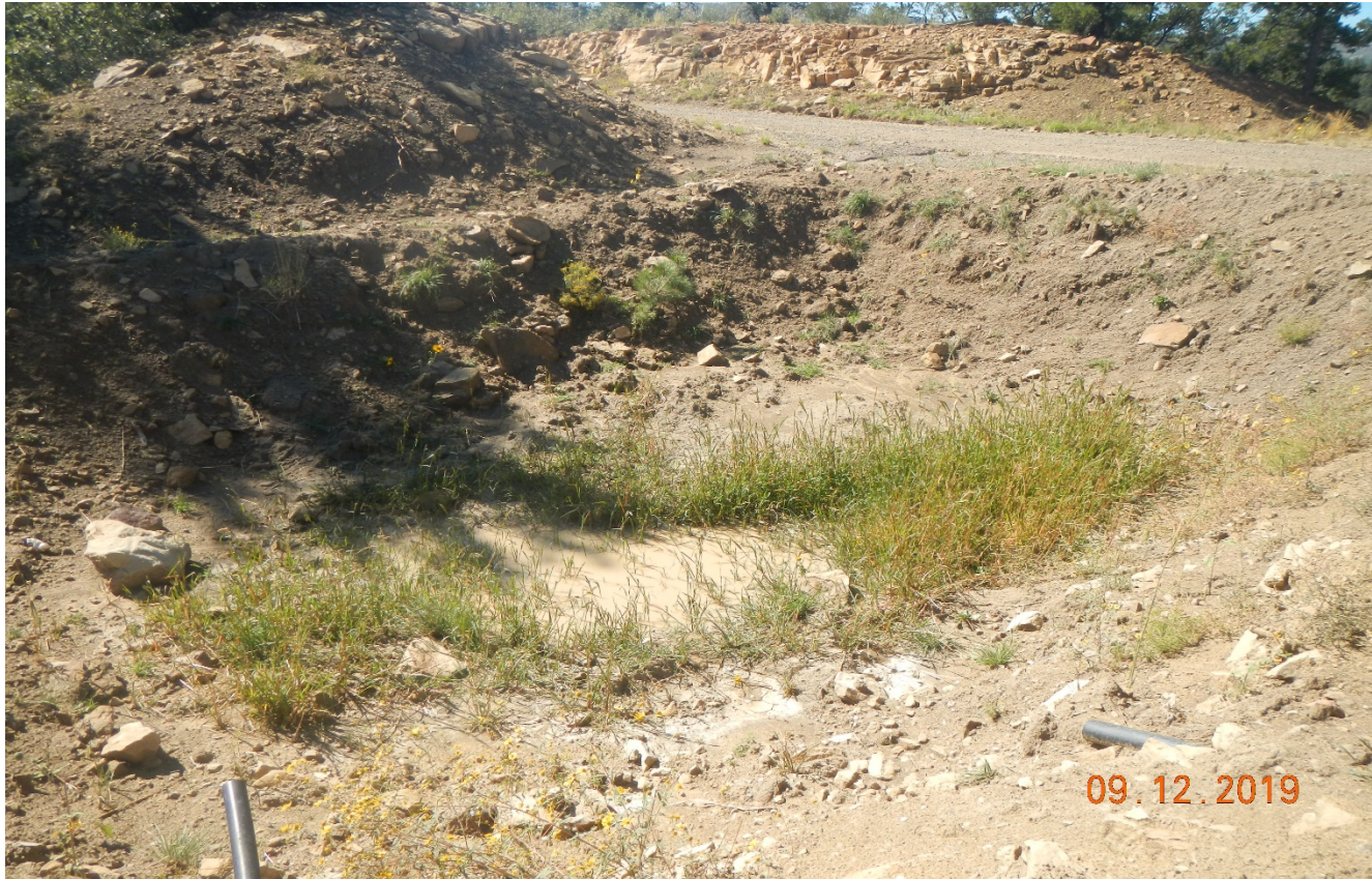
Photo 5. No freeboard marker was found in the pit. Corrective action of previous inspection not performed.
