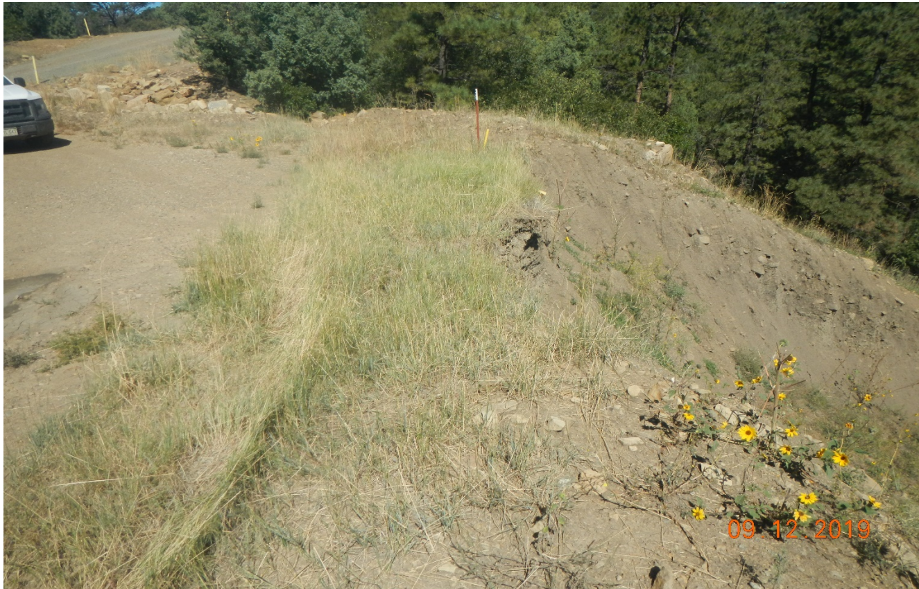
Photo 3. View of soil material that moved down the hill side.
