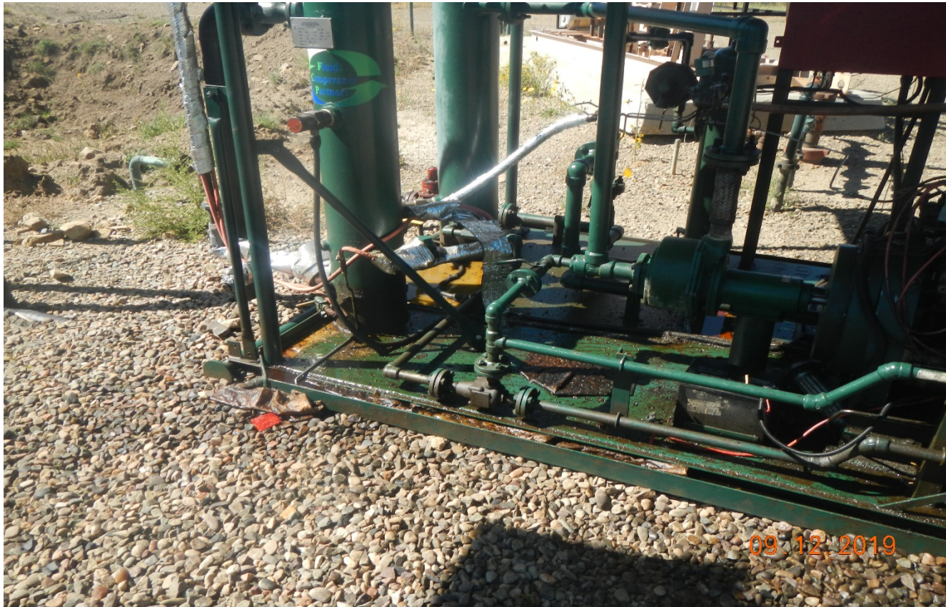
Photo 5. There is oily waste on the skid.
