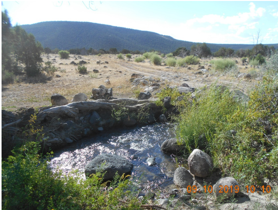
Access Road crossing irrigation ditch. Looking SE
