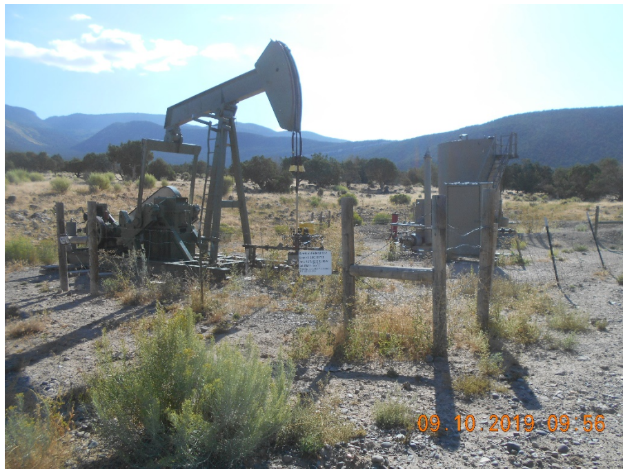
Wellhead with Pump jack, fencing and sign.
