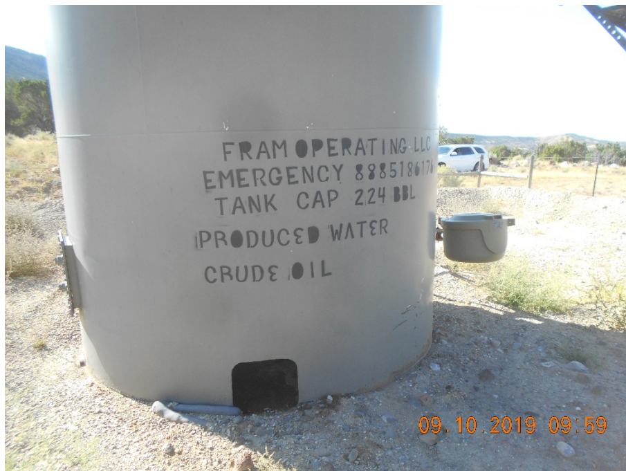
Tank battery label and inspection opening
