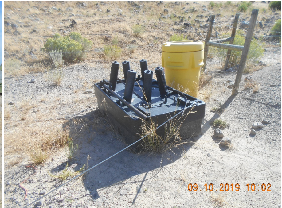
Spill response kit and chemical injector secondary containment (unused)
