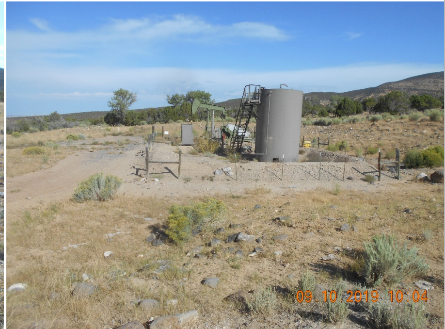
Location overview from SE corner looking NW.
