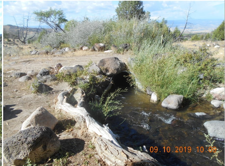
Culvert for irrigation ditch looking SW
