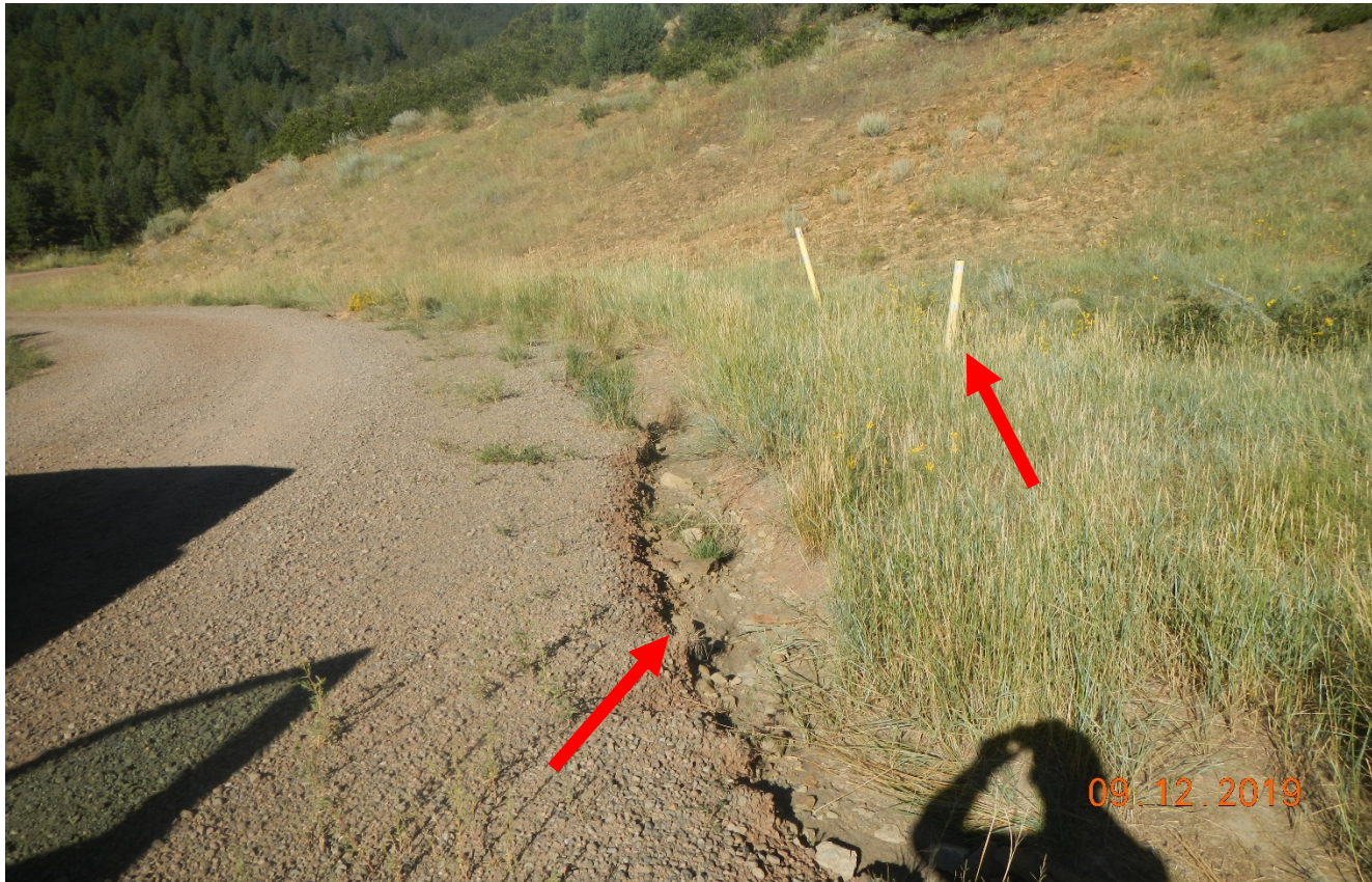
Photo 1. Stormwater is draining down the access road and not towards the culvert shown by red arrows.
