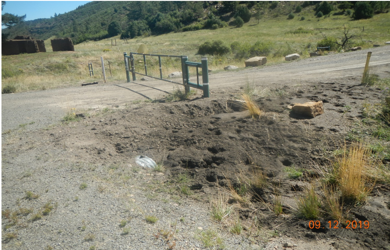
Photo 1. The culvert near the location has filled in with sediment. Erosion needs to be controlled from the source. Corrective action was not performed since previous inspection.
