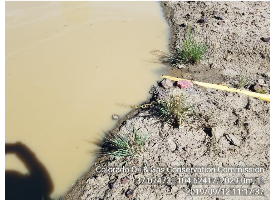
PHOTO 4: PRODUCED WATER LEVEL IN PIT IS ABOVE THE 2' FREEBOARD MARKER. SPOKE WITH JACK WISEMAN BY PHONE TO LOWER PIT LEVEL. Lower fluid level so at least two feet of freeboard exists per Rule 902.b.
