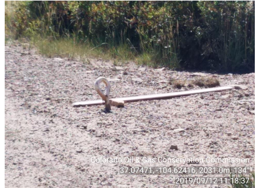
PHOTO 6: PHOTO 5: GUY LINE ANCHOR MARKER IS DOWN. Install proper guy line markers per Rule 1003.a
