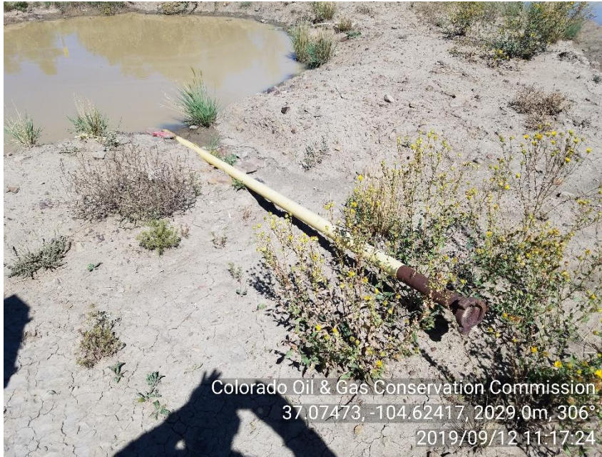
PHOTO 3: UNUSED EQUIPMENT 2" PIPE IN PIT. REMOVE UNUDED EQUIPMENT, COMPLY WITH RULE 603.f. CA DATE 10-12-19
