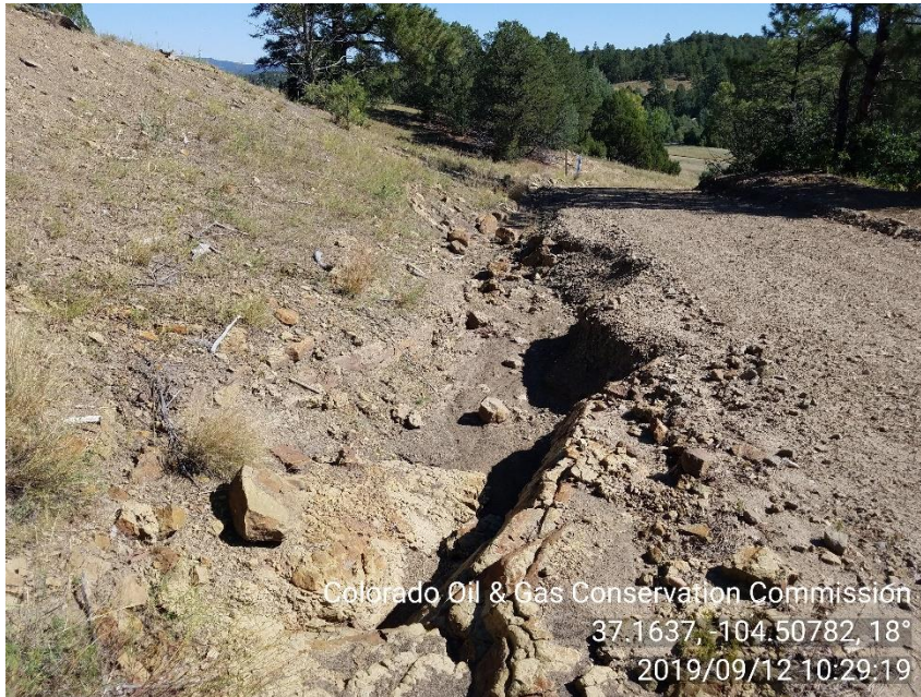
PHOTO 3: DITCH ON ROW NORTHEAST OF LOCTION IS ERODING NO BMP'S IN PLACE TO PREVENT DITCH FROM ERODING. REPAIR EROSION AND INSTALL BMP'S TO PREVENT MORE EROSION, COMPLY WITH RULE 1002.f. CA DATE 10-12-19
