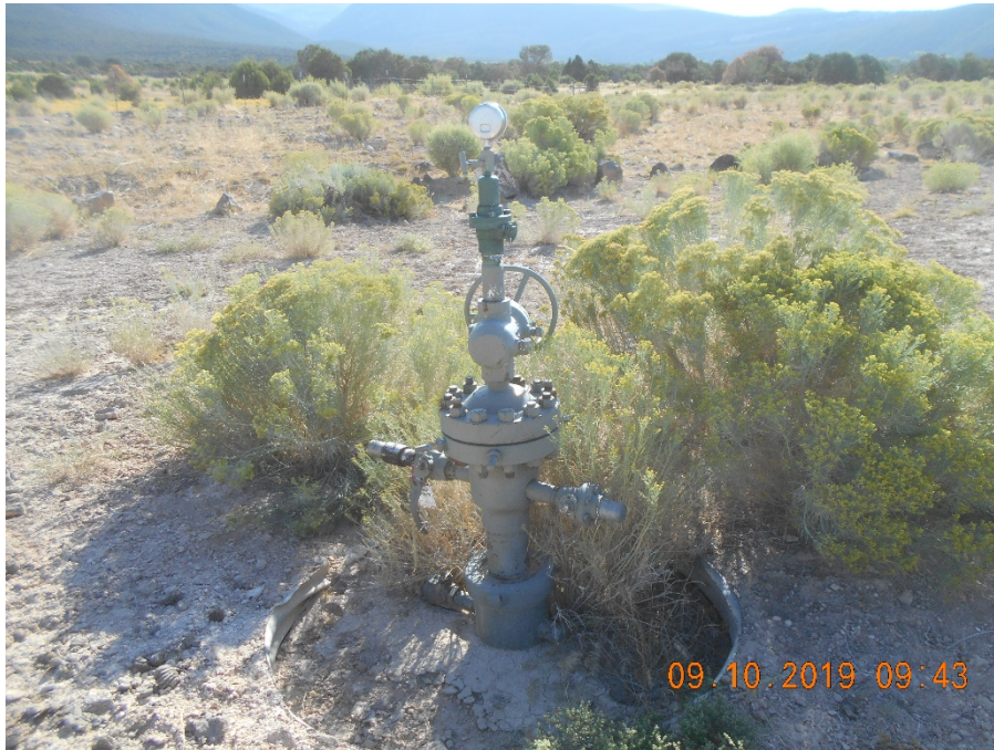
Wellhead looking E. Temporarily abandoned 150 psi on tubing gauge.
