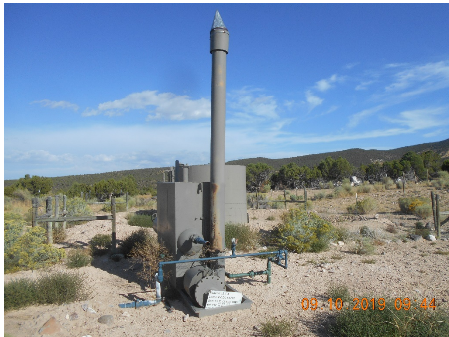
Separator with sign. Looking NW
