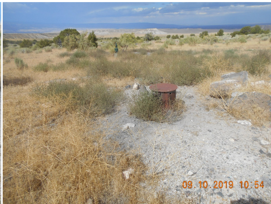
API # 05-077-09249 Lough #36-1-P 13 3/8" casing with welded plate (Sfc Csg / PA?) Looking W.
