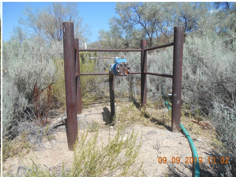
4" Gathering line riser. Green hose on ground is for private irrigation.
