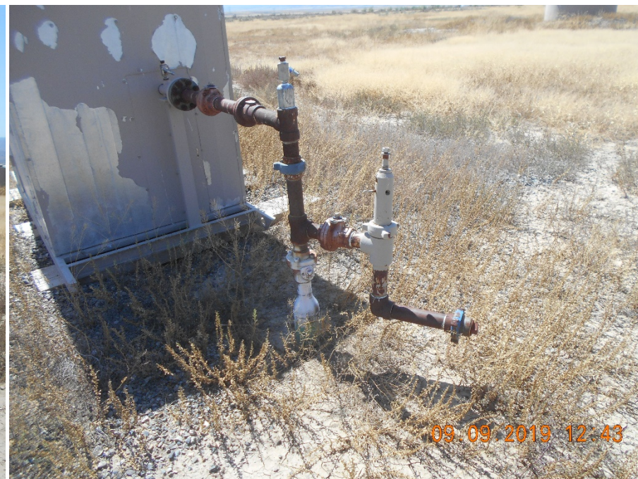
Meter housing to gathering line riser.
