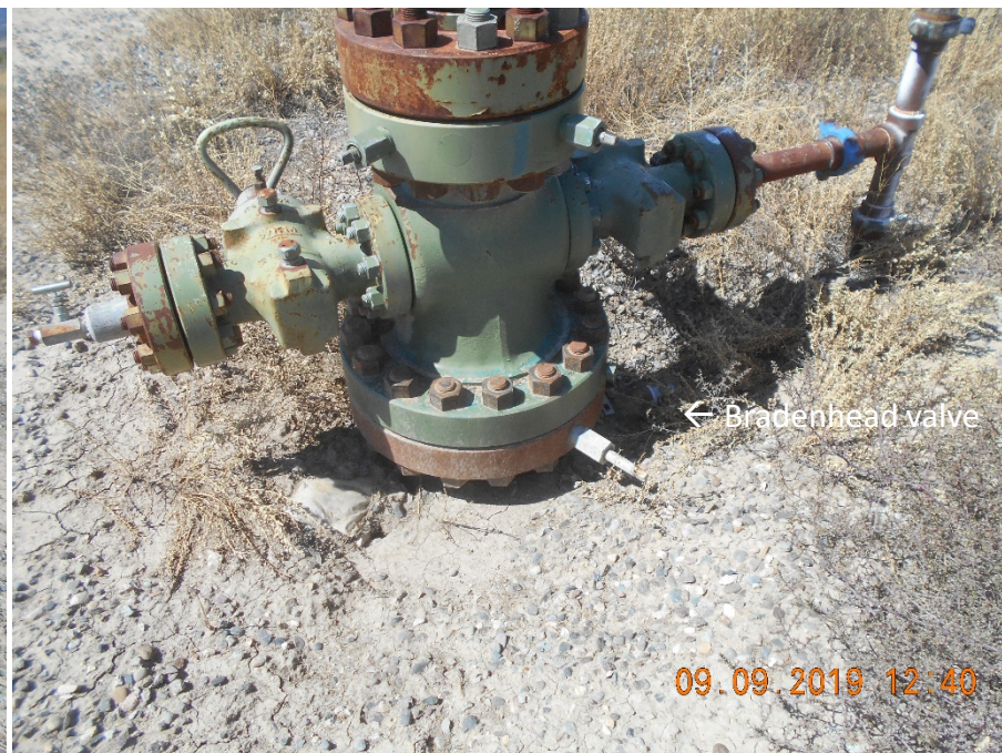
API # 05-077-09350 Whiting #26-5 wellhead with bradenhead valve exposed.
