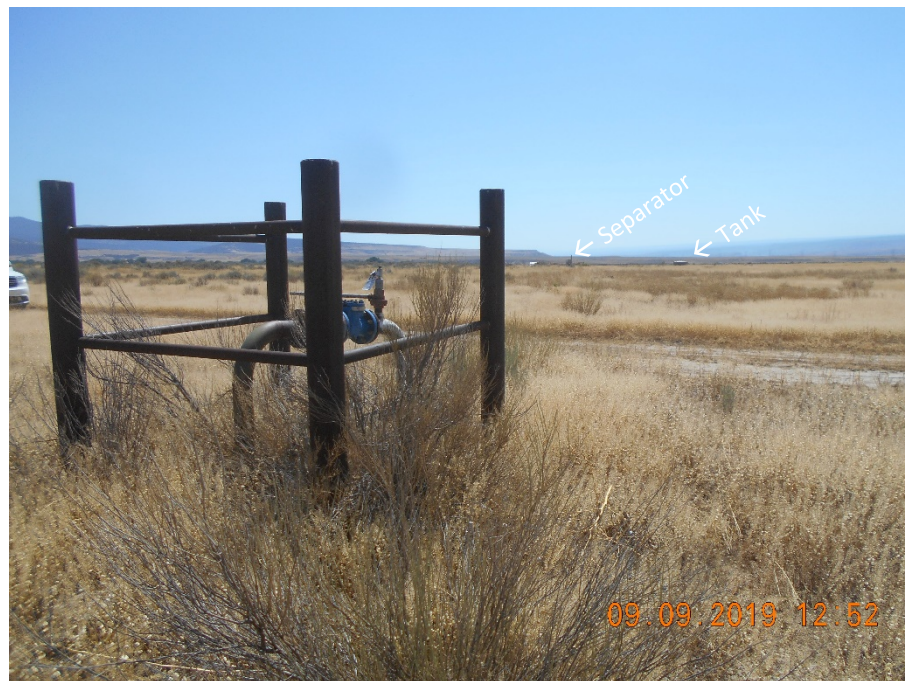
4" Gathering Line riser located ~ 680' NW of well. Looking SE
