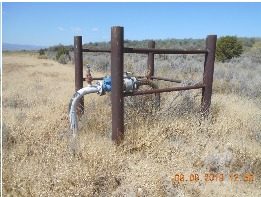
4" Gathering Line riser located ~ 680' NW of well. Looking W.
