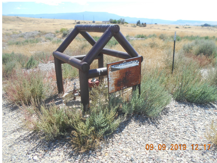
API # 05-077-09459 Kelly #23-2-B Wellhead with sign and pipe barricade looking SE Temporarily abandoned. Weeds,
