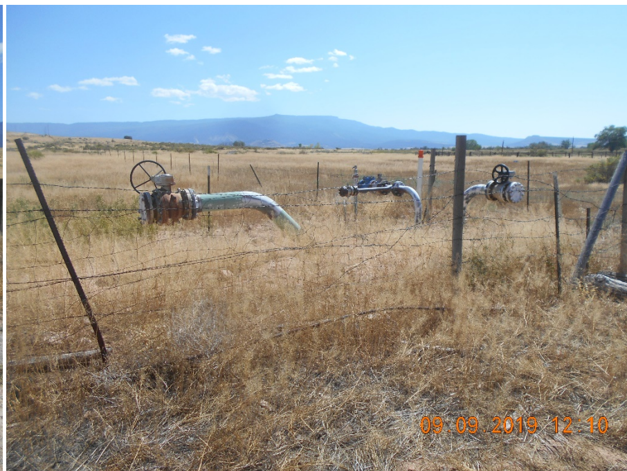
Gathering Line risers. 4", 6" & 8" Locked out/ tagged out with blind flange.
