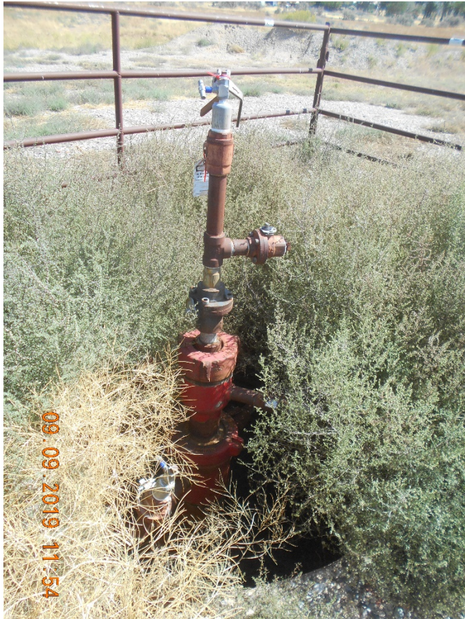
API #05-077-09314 Wellhead. Overgrown with weeds.
