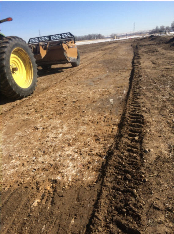
Removing road base 02/12/2019 1
