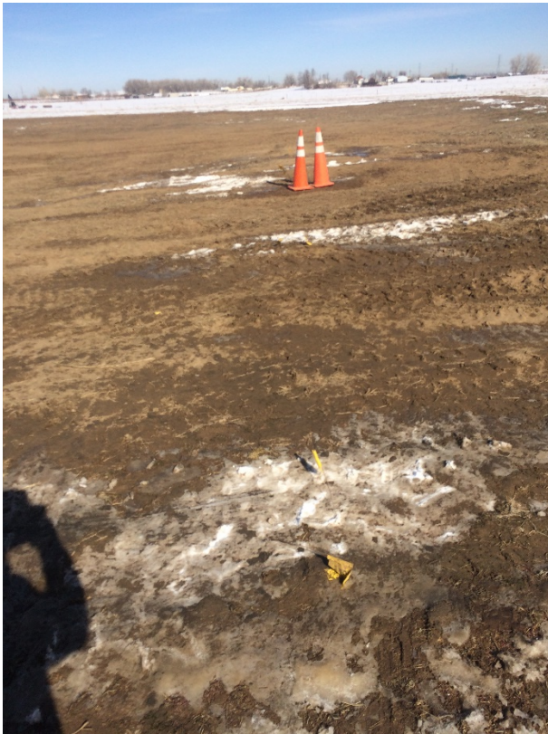
Potholing DCP Line 1
