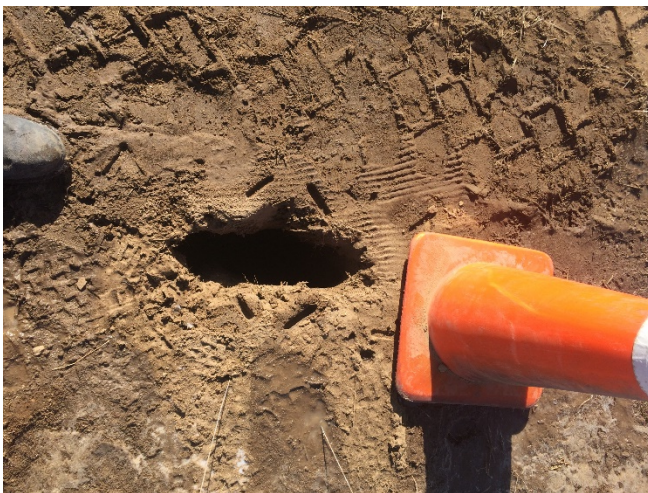
Potholing DCP Line 2
