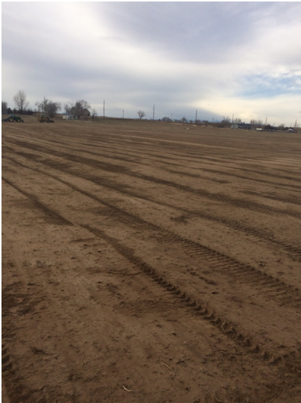
Final Grading of dirt work 1
